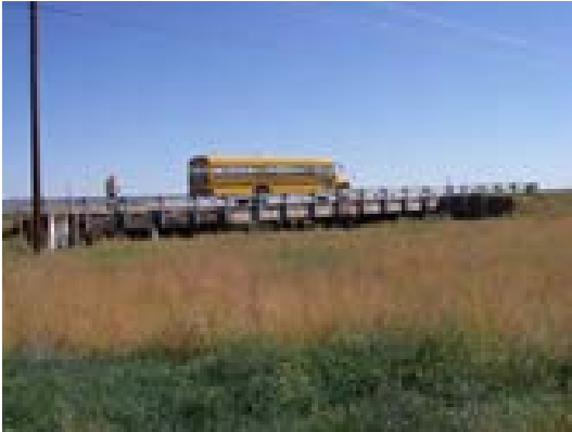
Figure 21: Bridge F-19-E Source: CDOT
