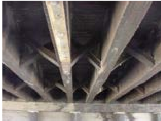
Figure 15: Bridge D-25-E– Concrete Collars to Reinforce Rotted Timber Supports Source: CDOT
