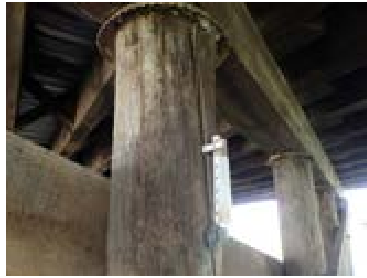
Figure 19: Bridge D-28-D – Split Timber Pile
