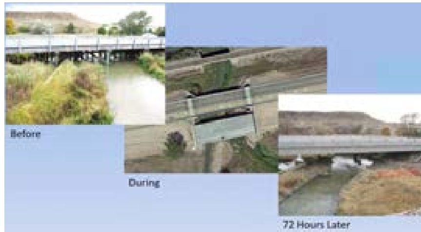
Figure 41: Use of Slide-In Method to Replace a Bridge Along US Route 34 (2013)
