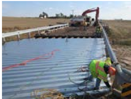
Figure 16: Bridge D-25-E – Deck Replacement Requiring Full Closure Source: CDOT
