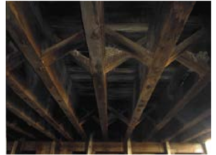
PHOTO OF EXISTING TYPICAL SECTION
