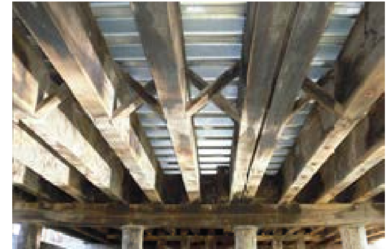
PHOTO OF EXISTING TYPICAL SECTION
