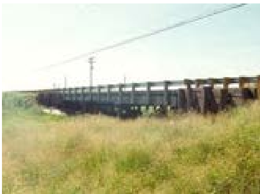
Figure 16: Bridge D-28-C Source: CDOT
