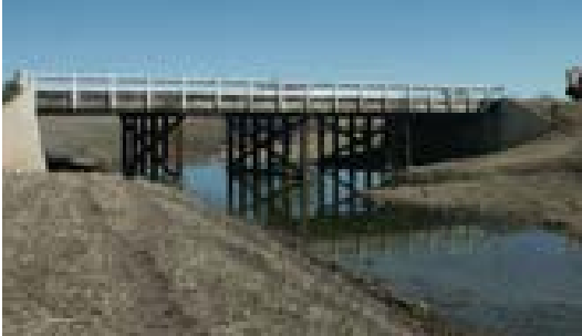
Figure 35: Bridge G-21-A Source: CDOT
