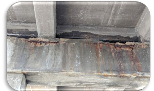
Deteriorated Pier Cap and Bearing Loss at F-20-BB
