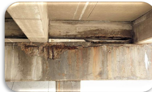
Deteriorated F-20-BA Pier Cap
