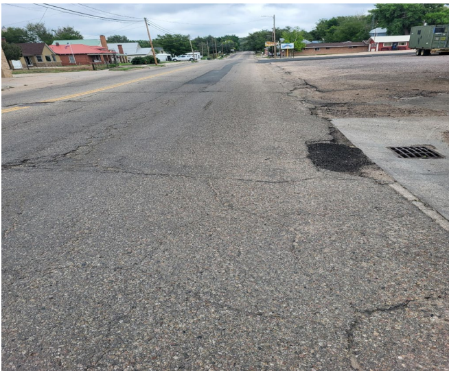
Compromised storm sewer with patch
