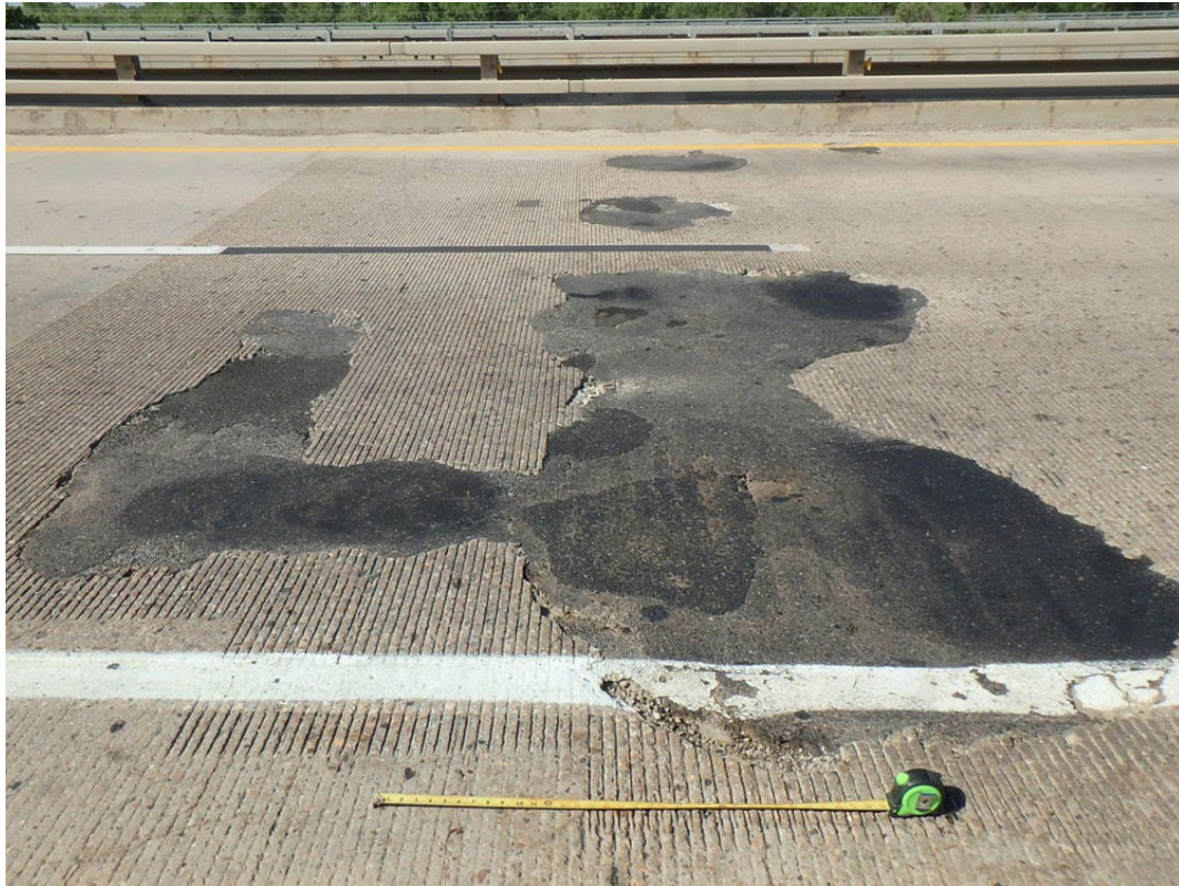
F-20-BJ: I-70 over Middle Bijou Creek. Failing Bridge Deck patch, typical deck condition throughout length of structure.
