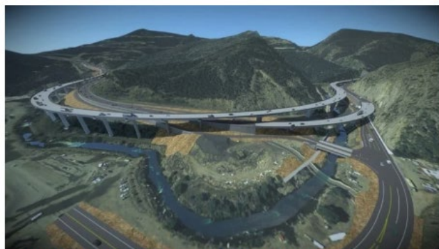
Rendering of the completed I-70 Floyd Hill Project I-70 alignment looking south, with westbound I-70 braiding over eastbound I-70 at the bottom of Floyd Hill.
