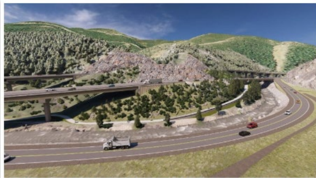
Design rendering of the new I-70 Floyd Hill Project highway alignment, facing south. Pictured from top to bottom: westbound I-70, eastbound I-70 and the new US 6 frontage road that connects to the Hidden Valley/Central City Parkway (Exit 243) interchange.
