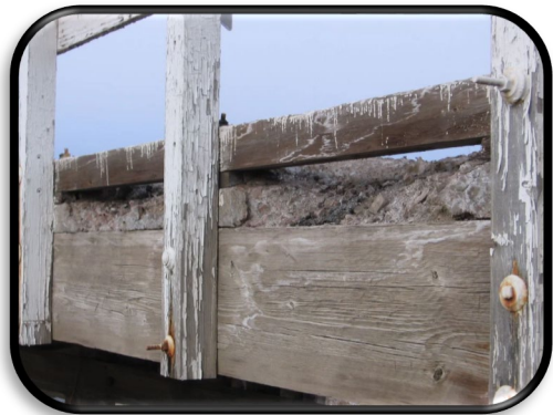
Deterioration and spalling of edge of deck on F-19-C
