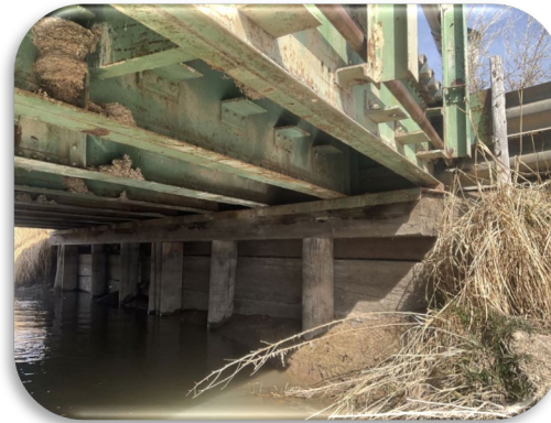
Girders and abutment at J-04-X
