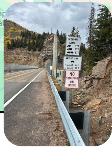
Load posting sign at Red Cliff Arch
