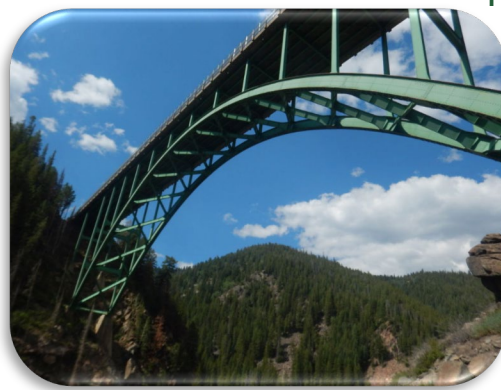
Underside looking south Red Cliff Arch
