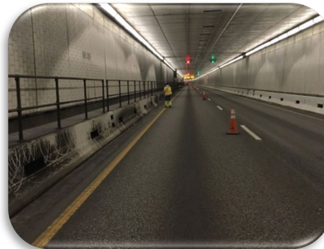
Lighting in EJMT during inspection
