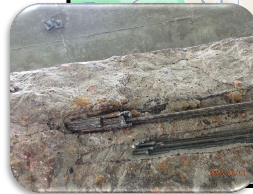
Broken PT strands in girder at C-22-AY
