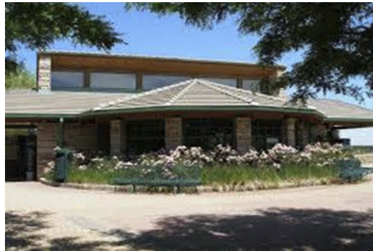
Colorado City Exterior flatwork repairs & new HVAC
