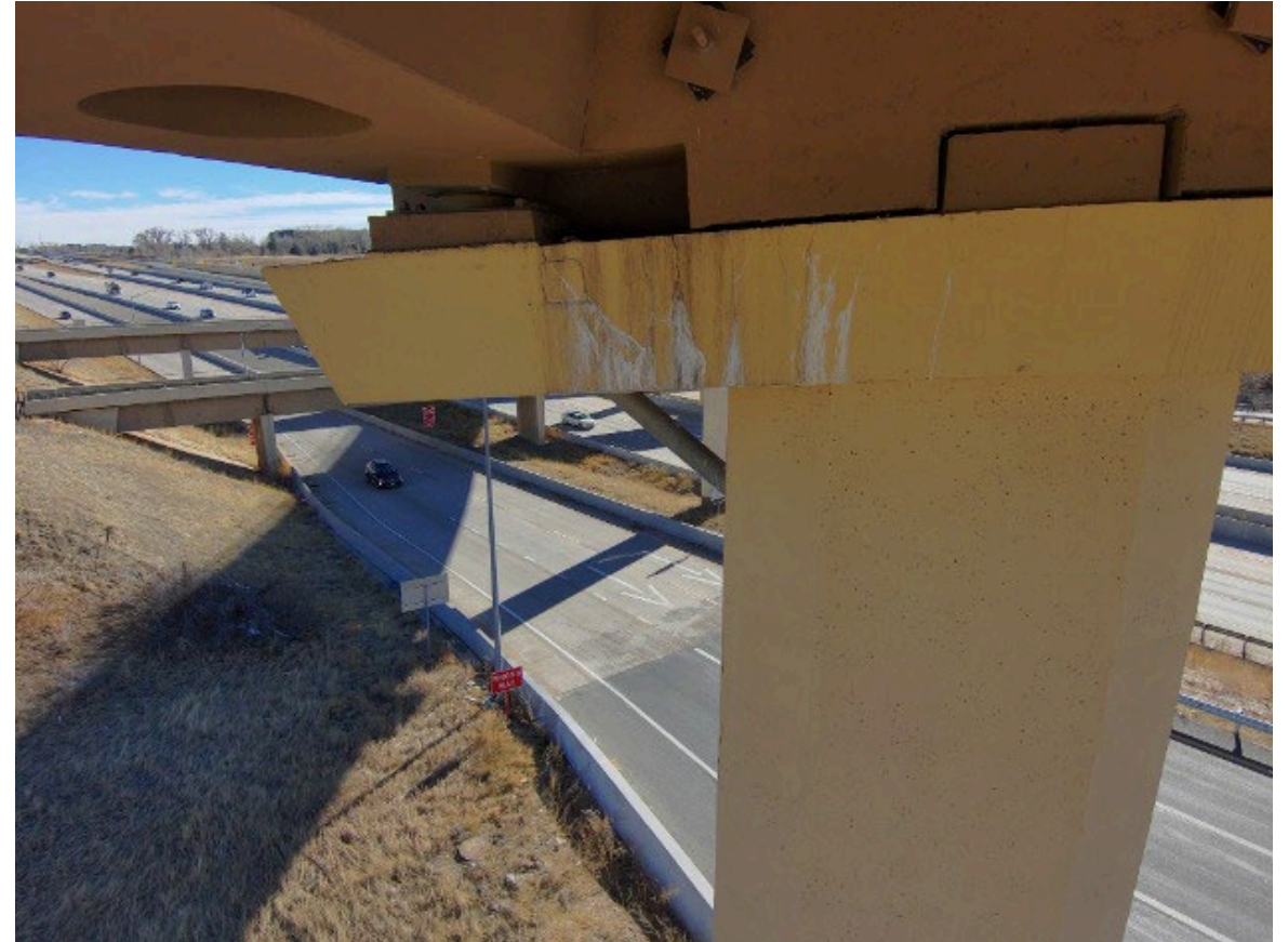
Pier 7: North Face of Pier Cap
