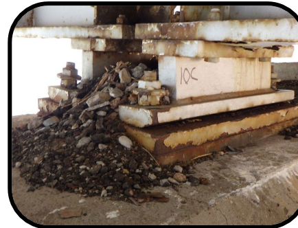
Heavy Debris, Surface Rust, and Paint System Failure at a Bearing
