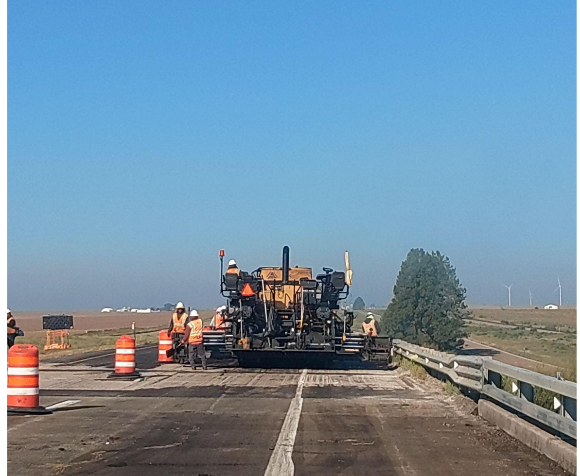
Structure G-28-N on I-70
