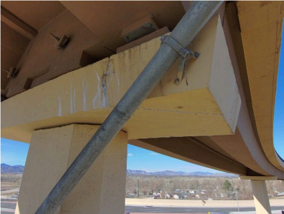
Pier 7: South Face of Pier Cap
