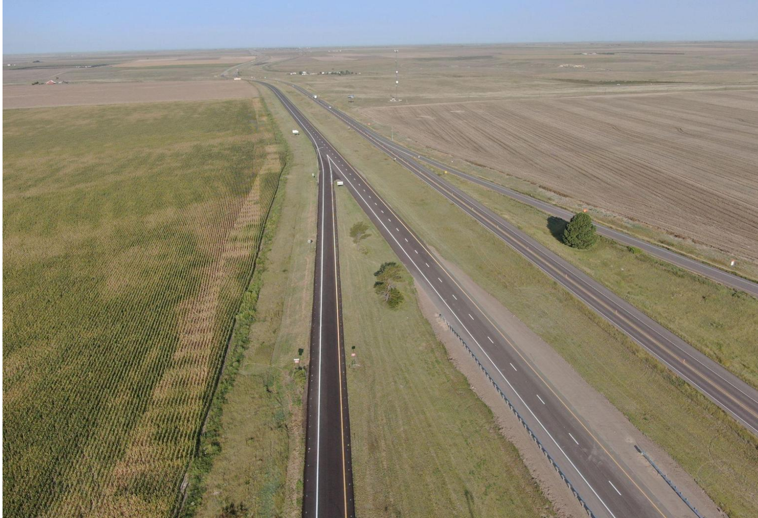
Bethune Interchange looking westbound
