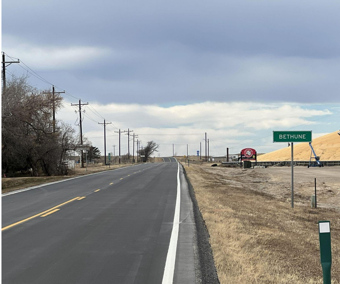
US 24 Bethune looking West
