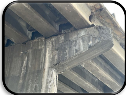
Pier with exposed rebar and delamination at E-17-IE
