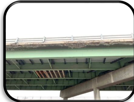
Exposed corroded rebar on overhang of E-17-IJ
