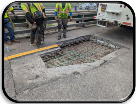
Deck repair patch on E-17-IF
