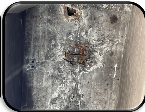
Spall and delamination with exposed rebar in bay of F-16-DA
