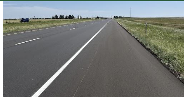
I-70 Improvements near Kansas
