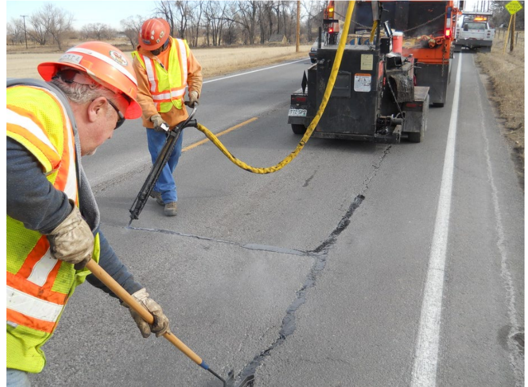
Crack sealing Hwy 7 pt 13 1-24-13
