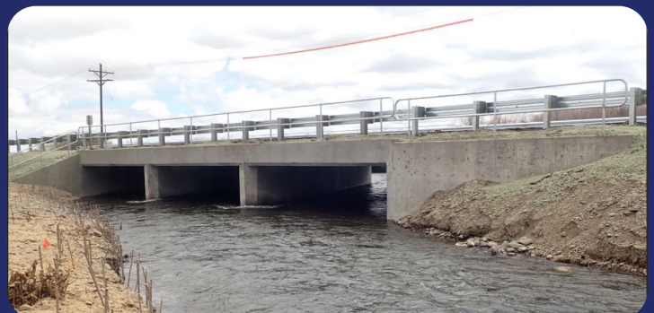
US 285 over Conejos River Overflow | Region 5 | Conejos County
