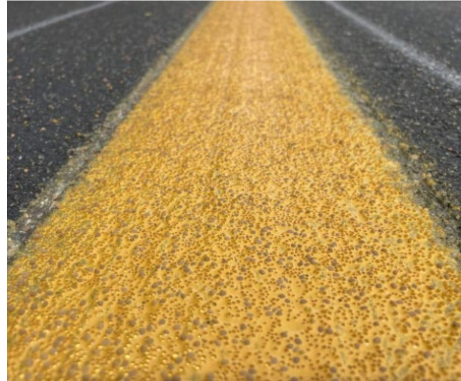
Epoxy Pavement Marking
