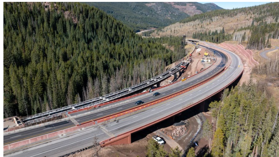
I-70 West Vail Pass Auxiliary Lanes Project eastbound I-70 new bridge aerial view.
