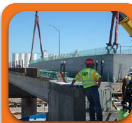
April 27, 2018: Construction Begins
