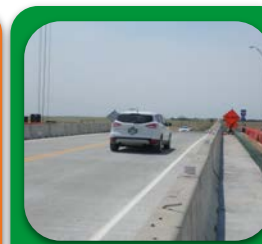
June 29, 2018: Bridge is Open to Traffic
