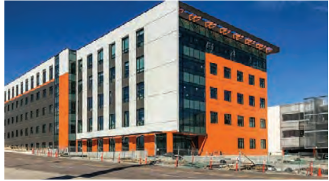
CDOT's Headquarters (above), in the Sun Valley neighborhood, replaced CDOT's former headquarters building and Region 1 offices in 2018.
