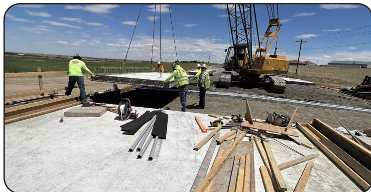
Image 21 & 22. Bridge Deck Rebar and Pre-cast Bridge Approach Installation on US 36 ML over Draw (F-19-E)
