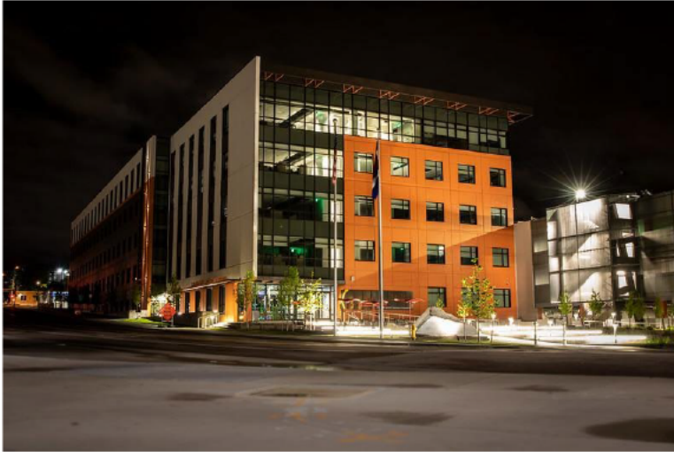
CDOT HQ Building
