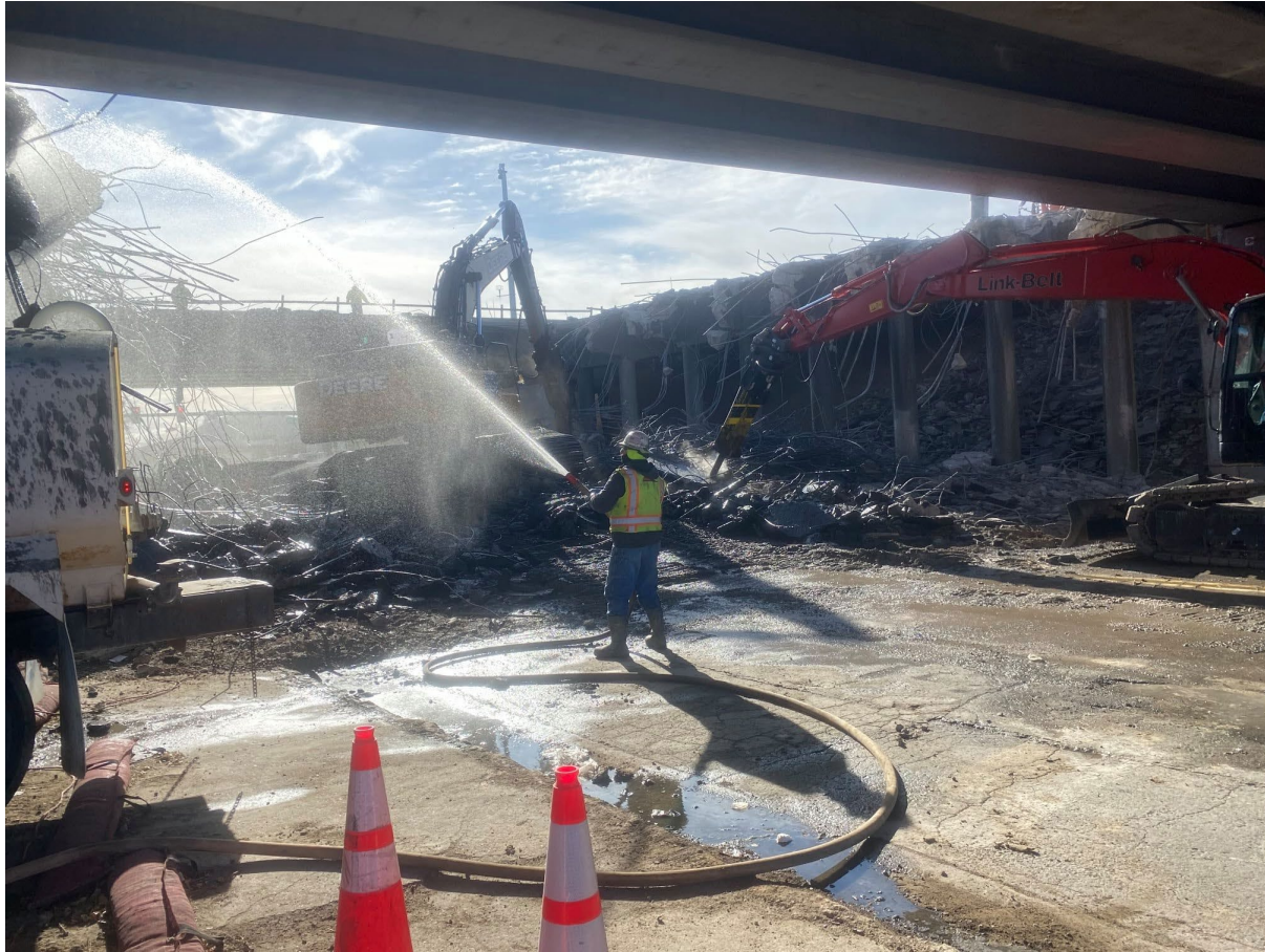
Caption: Dust mitigation during the viaduct demolition as part of the Project's robust environmental protection efforts.
