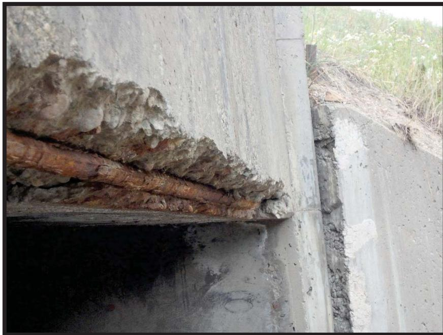
**Photo 26 Bottom edge of top slab at south end, major spalling with exposed rebar along entire edge**
