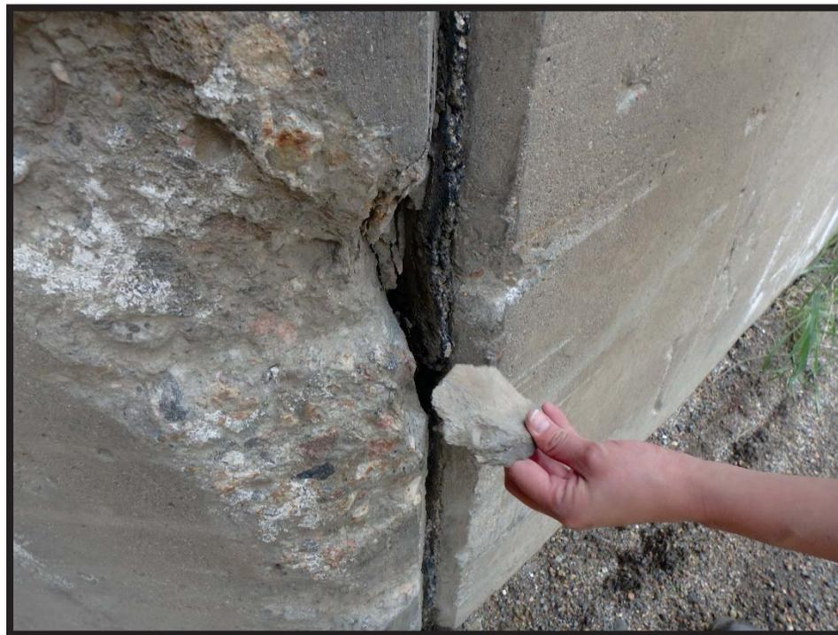
**Photo 5 NW Wingwall at culvert joint, significant spalling**
