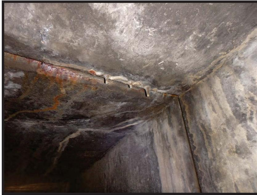
**Photo 15 East Wall/Top Slab at construction joint 53-ft from North. Actively leaking and showing stalactites, efflorescence, delamination**
