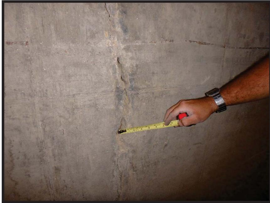
**Photo 19 West Wall at 50-ft from south, showing vertical 1/2 to 3/4-inch shear crack**
