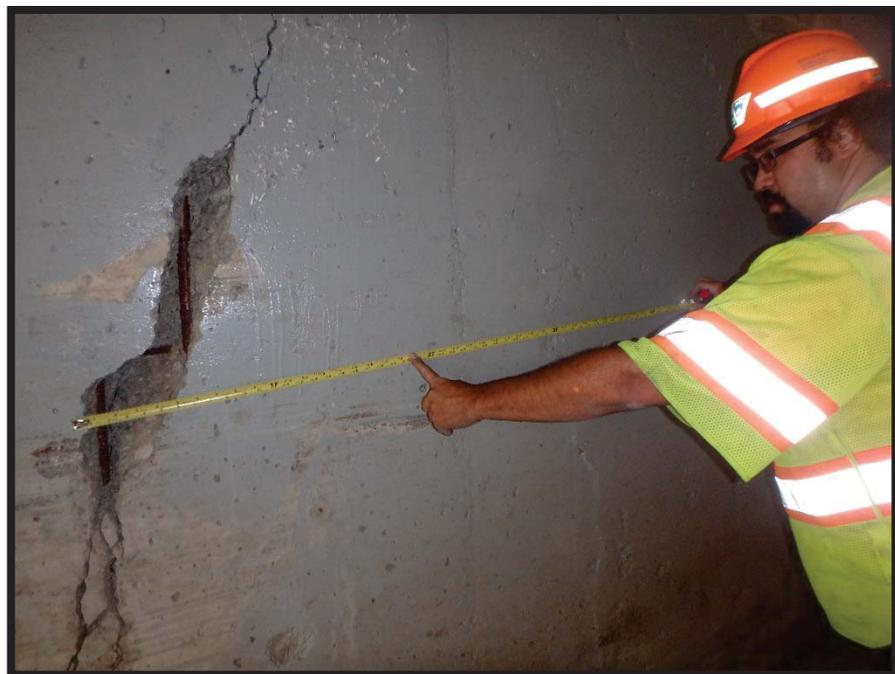
**Photo 22 West Wall at 22-ft from south, showing diagonal shear crack ranging from 1/8 to 4-inches, migrating from top to bottom, spalling**
