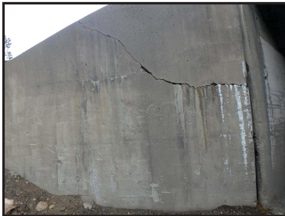
**Photo 6 NE Wingwall, 1 diagonal crack extending from top to culvert joint, other vertical and horizontal sealed cracks migration**
