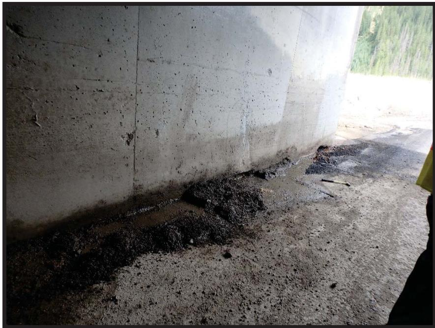
**Photo 24 East Wall at south end showing concrete deterioration and section loss at bottom for several feet, heaving leakage**
