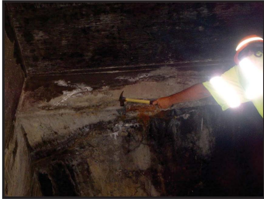
**Photo 17 Top Slab at 90-ft from North (EB median), showing efflorescence, delamination, unsound and spalling, and large crack migration throughout entire top slab down through wall**
