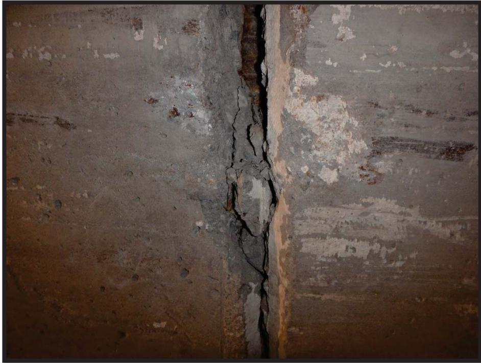
**Photo 13 West wall at 44-ft from north, spalled and exposed rebar**
