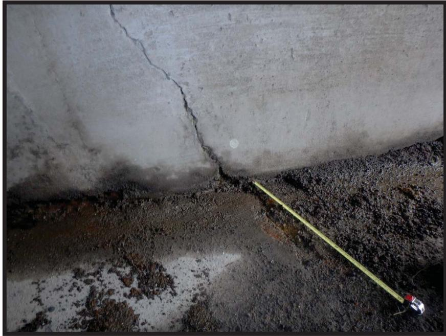
**Photo 23 East Wall at 22-ft from south, showing diagonal shear crack ranging from 1/8 to 4-inches, migrating from wall into bottom slab**
