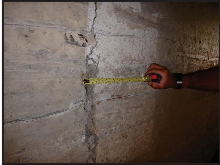
**Photo 21 West Wall at 48-ft from south, showing multiple migrating cracks varying between 1/8 to 2-inches**
