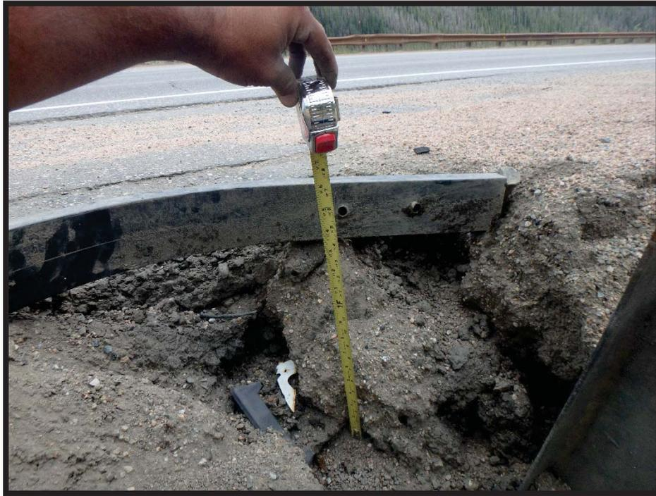
**Photo 1 WB shoulder at guardrail, erosion 15-inches deep**
