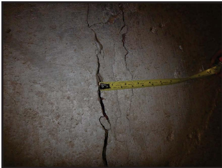
**Photo 20 East Wall at 55-ft from south, showing 2-migrating cracks varying 1/8 to 1/2-inch and spalling**
