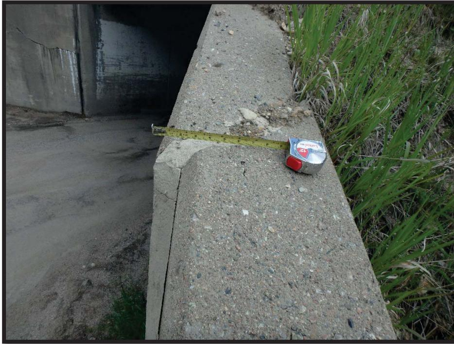
**Photo 3 NW Wingwall showing sealed fracture, 4-iches of displacement**
