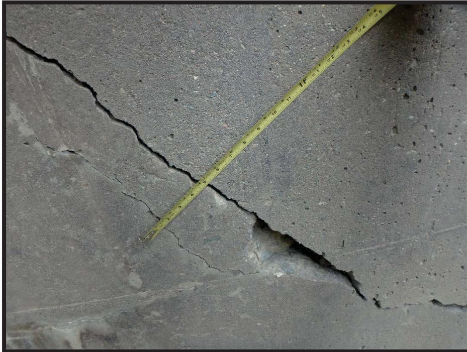
**Photo 7 NE Wingwall, showing 3/8 to 1/2-inch crack with spalling in between migrating smaller crack, refer to photo 6**
