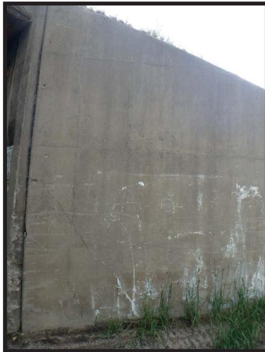
**Photo 4 NW Wingwall showing diagonal 1/8-inch crack extending from joint to bottom**
