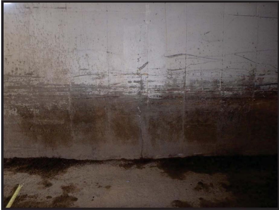
**Photo 11 West wall, vertical 1/4-inch shear crack migrating from top to bottom located at 26-ft from north end**
