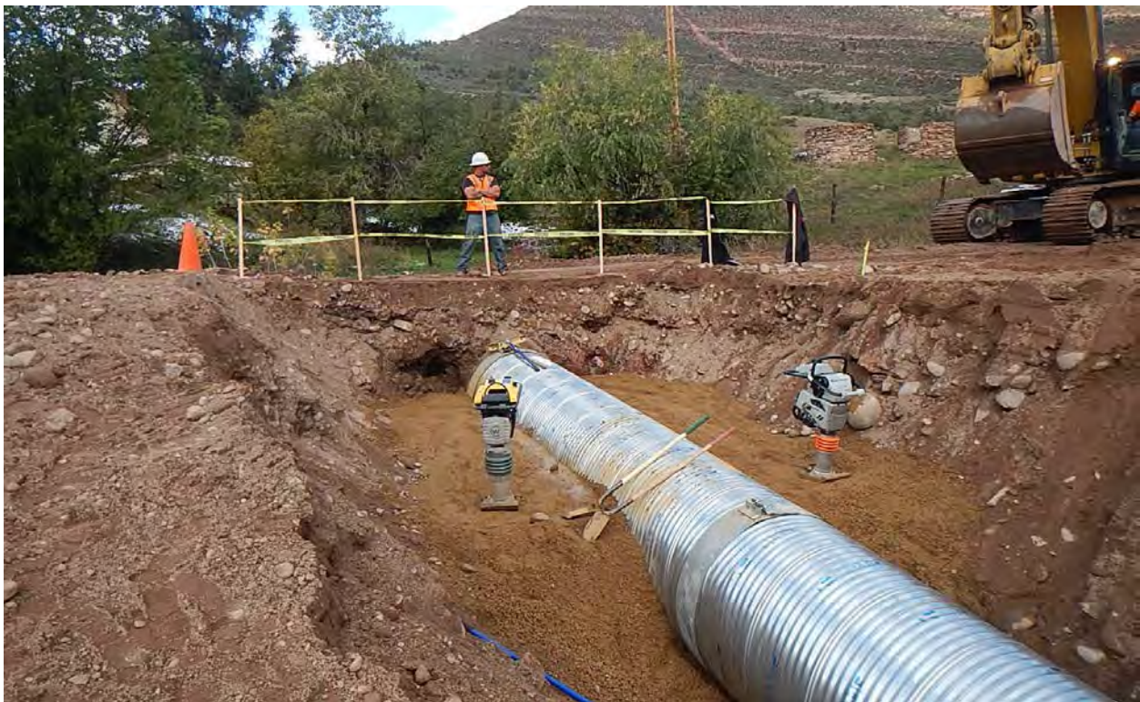
Figure 71 - MP 31.2, ER CMP Installation.
