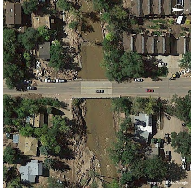
Figure 75 - MP 32.98 Pre-disaster aerial photo
