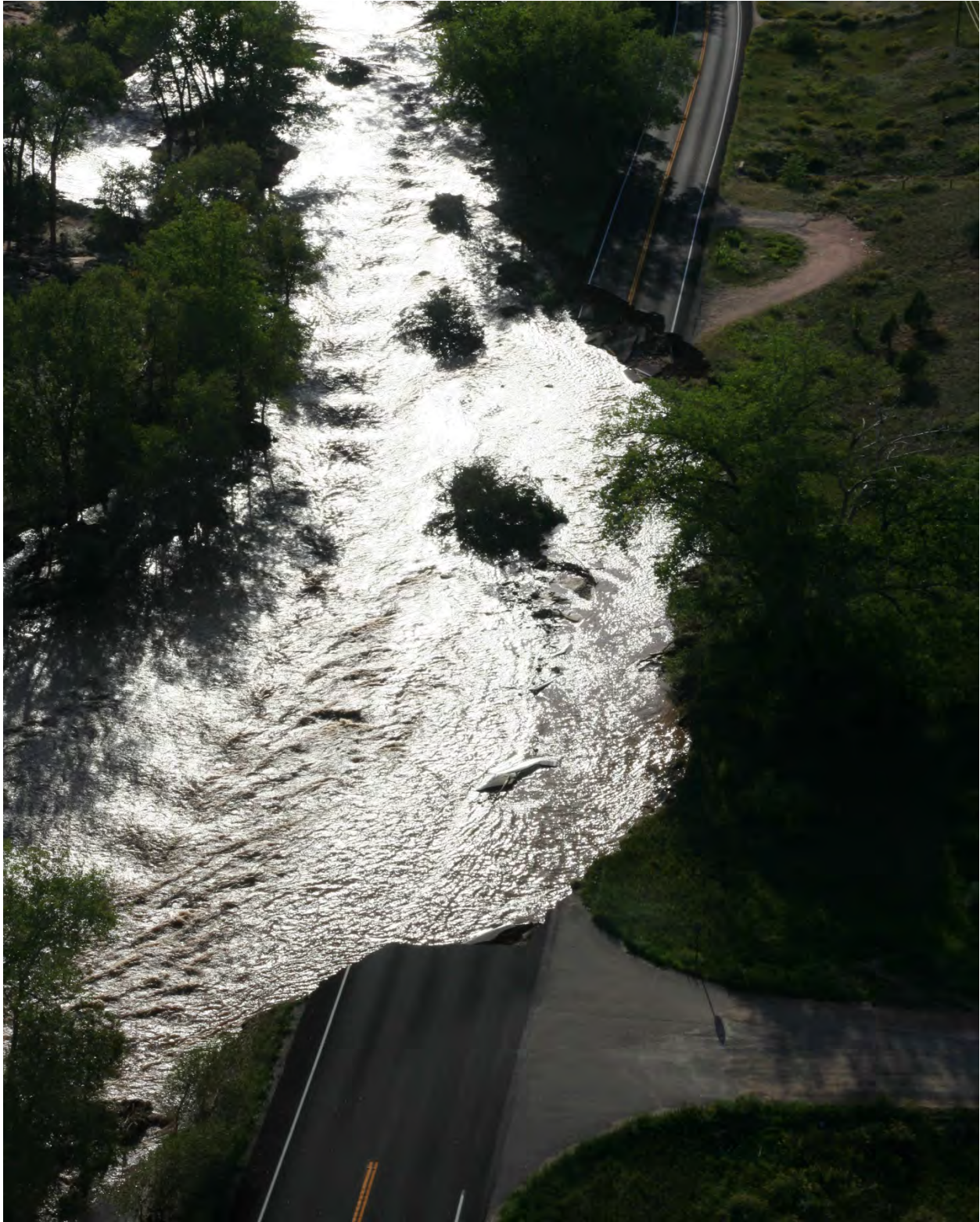
Figure 64 - MP 31.64, Complete loss of roadway.
