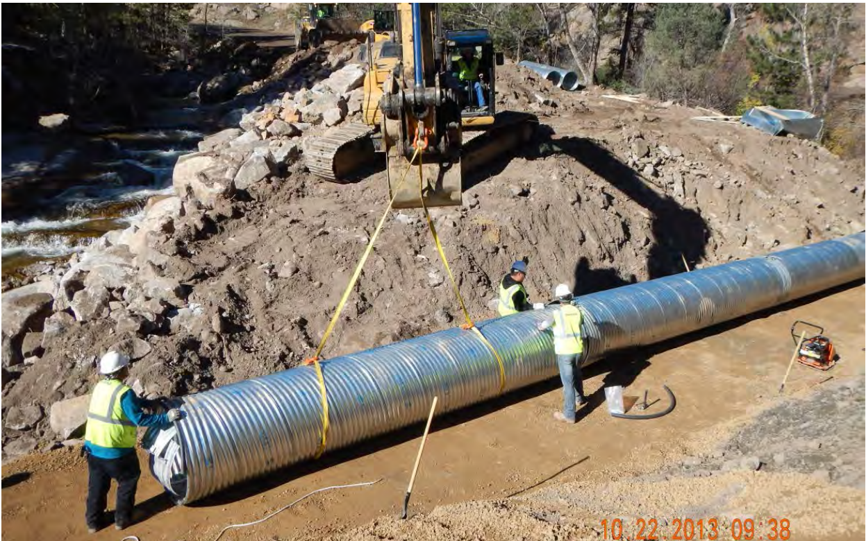
Figure 48 - MP 23.8 Facing northwest, CMP repair.
