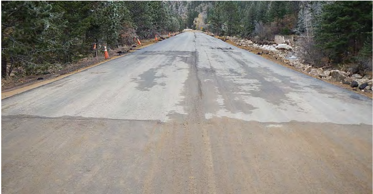
Figure 45 - MP 23.4 Facing east, Completed ER roadway section.
