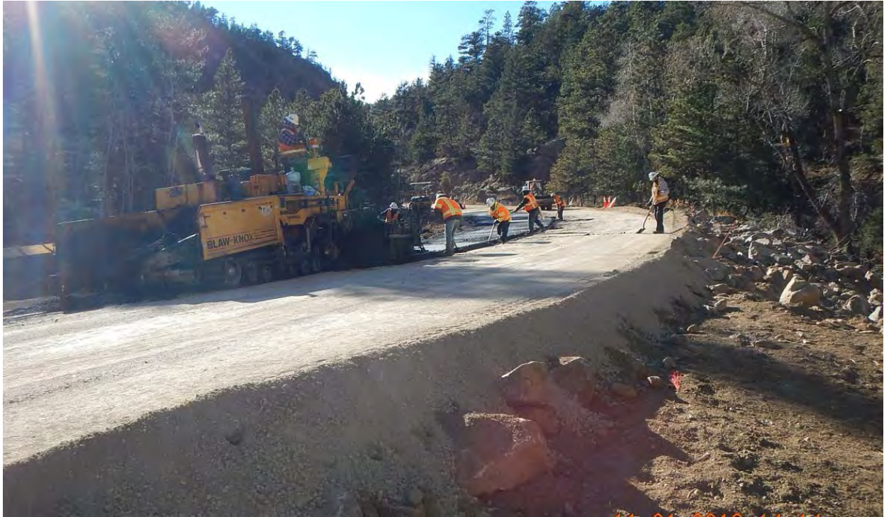
Figure 47 - MP 23.8 Facing west, Roadway repair.
