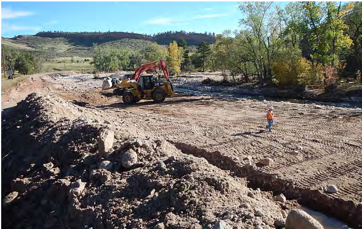
Figure 67 - MP 31.2, Facing southwest, ER Roadway repairs.
