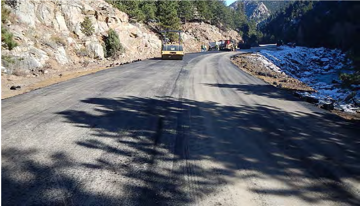
Figure 51 - MP 25.5 Facing east, Roadway repair.
