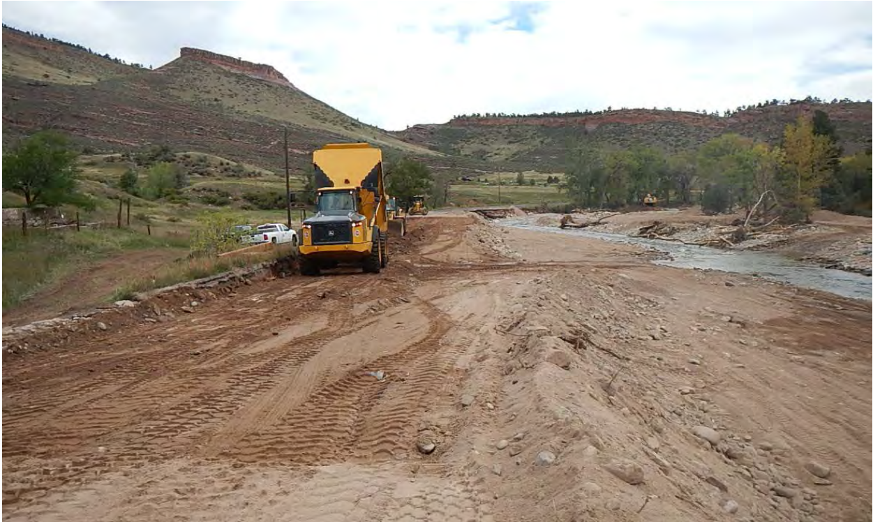
Figure 68 - MP 31.2, Facing northeast, ER Roadway repairs.
