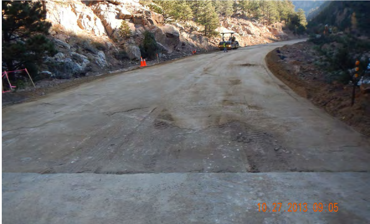
Figure 49 - MP 24.7 Facing northeast, Roadway repair.
