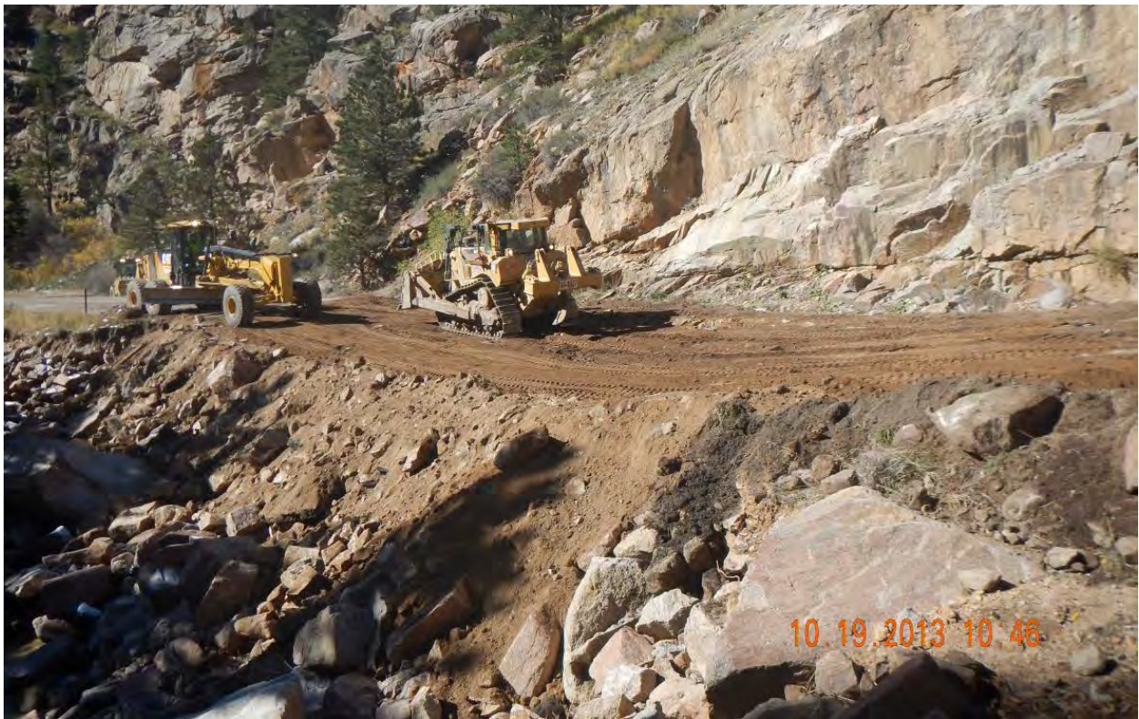
Figure 52 - MP 25.9 Facing west, Roadway repair.
