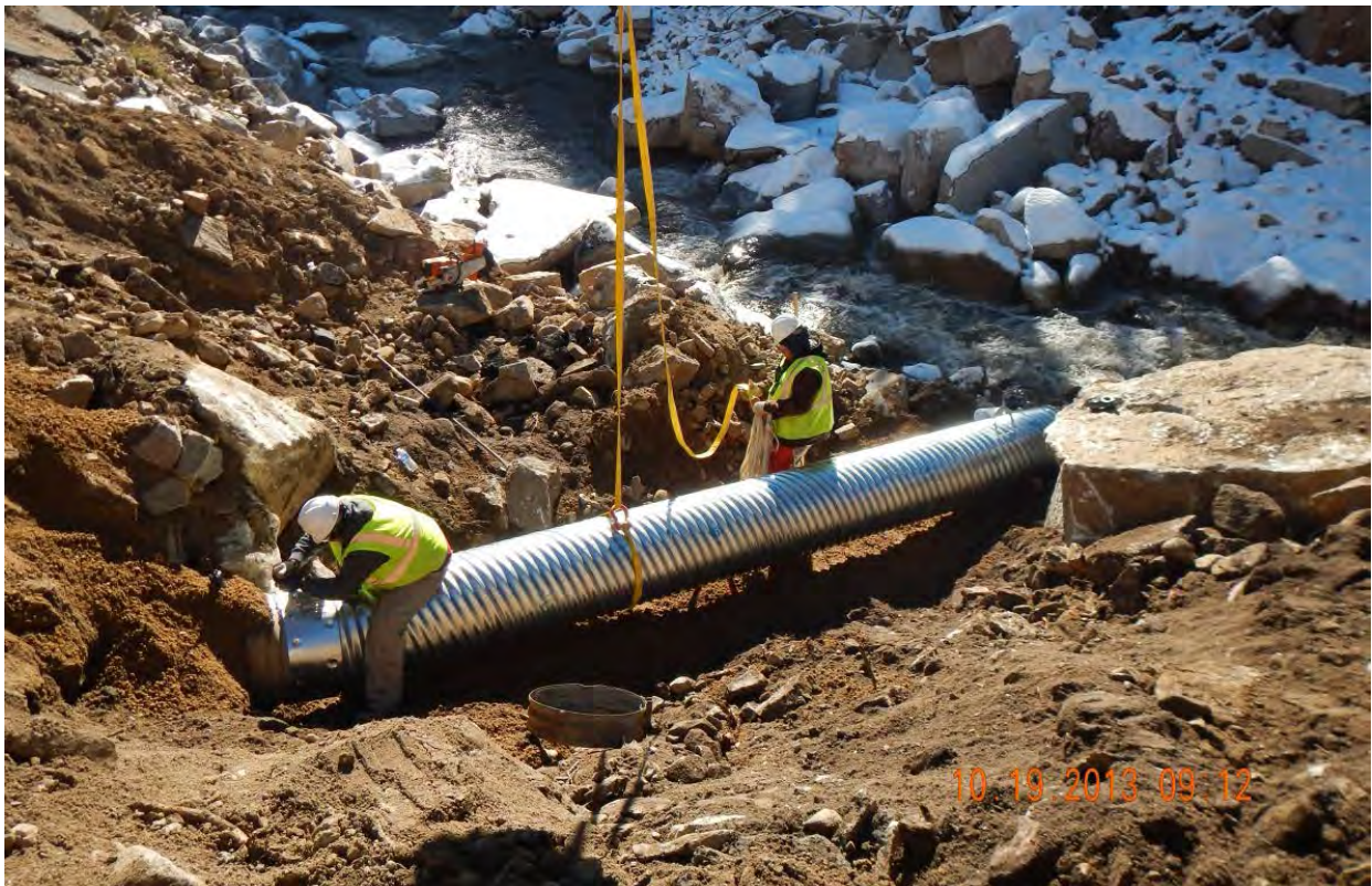
Figure 46 - MP 23.4, CMP repair.
