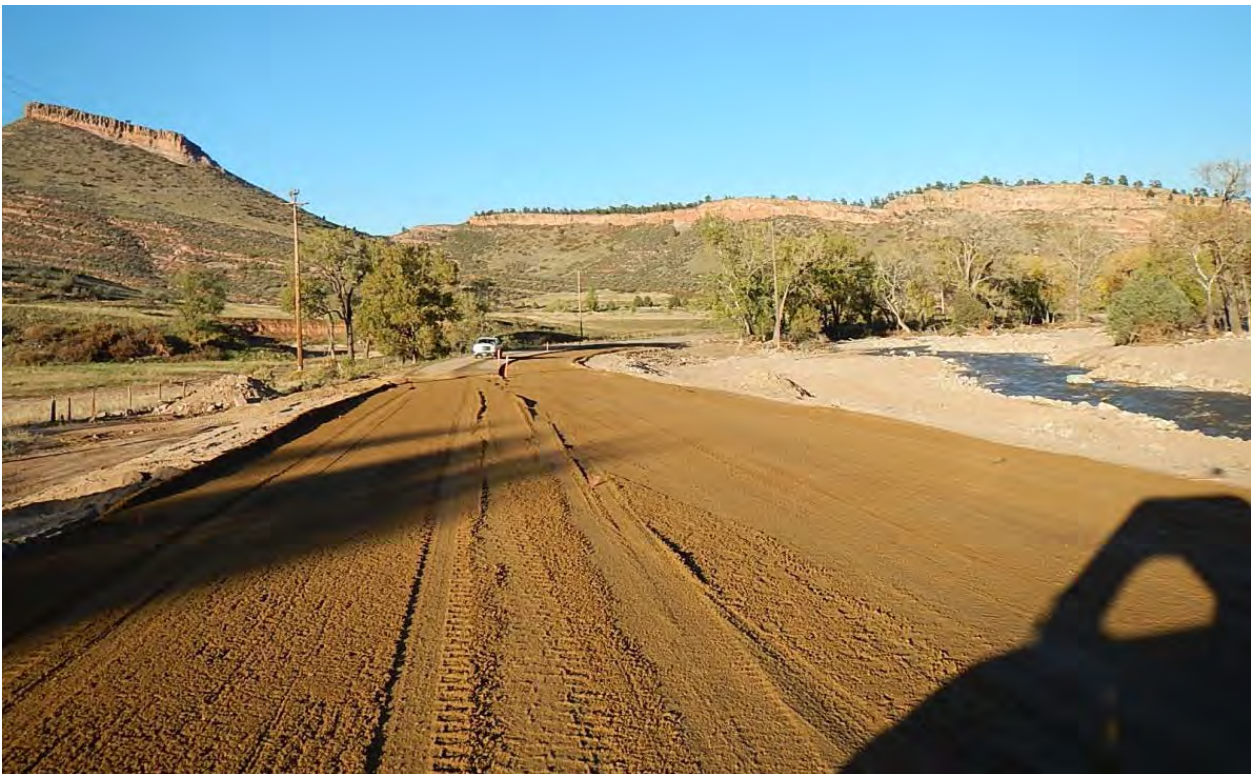
Figure 69 - MP 31.2, Facing northeast, ER Roadway repairs.
