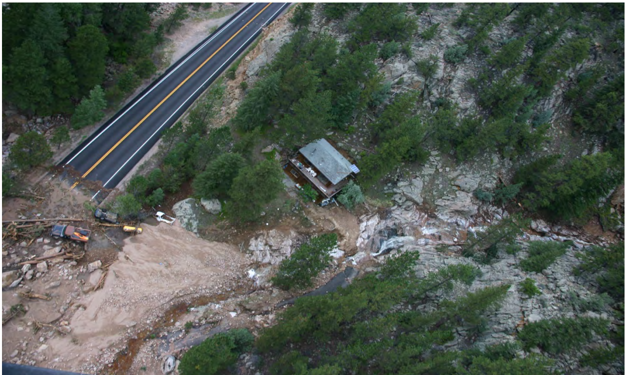
Figure 27 - MP 24.6, Rock slide, debris and sediment covering both roadway lanes.
