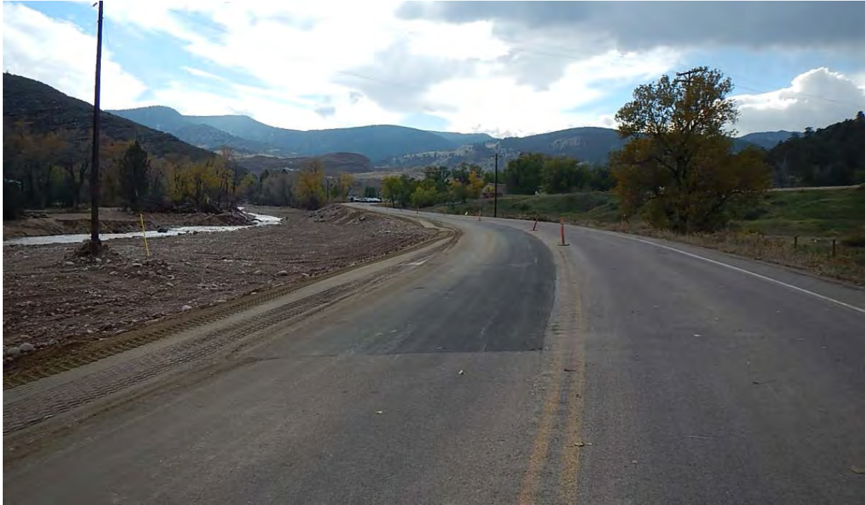
Figure 70 - MP 31.2, Facing southwest, ER Roadway repairs.
