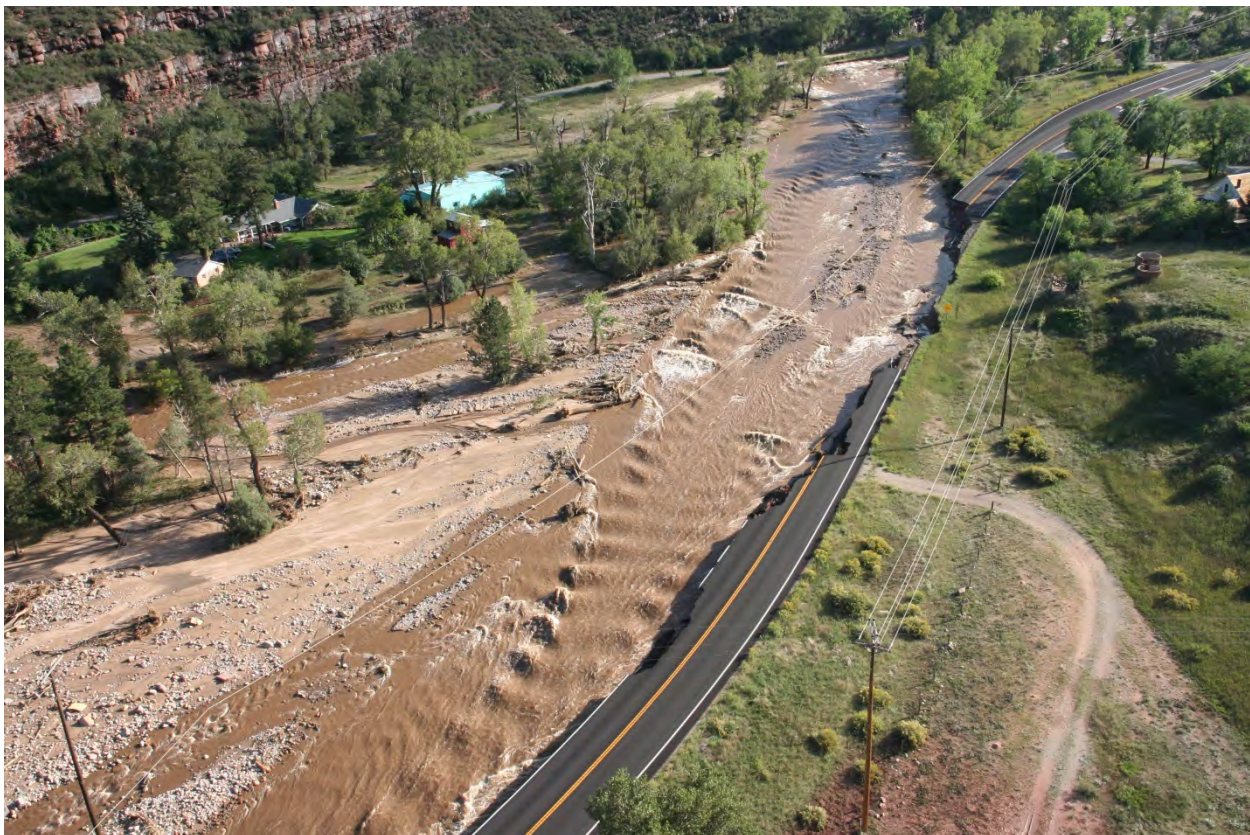
Figure 63 - MP 31.3 – 31.42, Riverside embankment washout and EB and WB undermined pavement loss.
