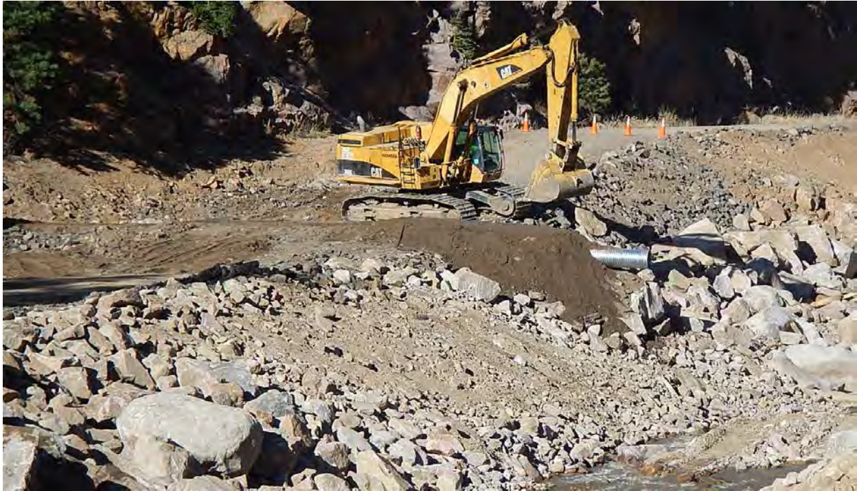
Figure 57 - MP 27.2, Facing north, Roadway and CMP repair.
