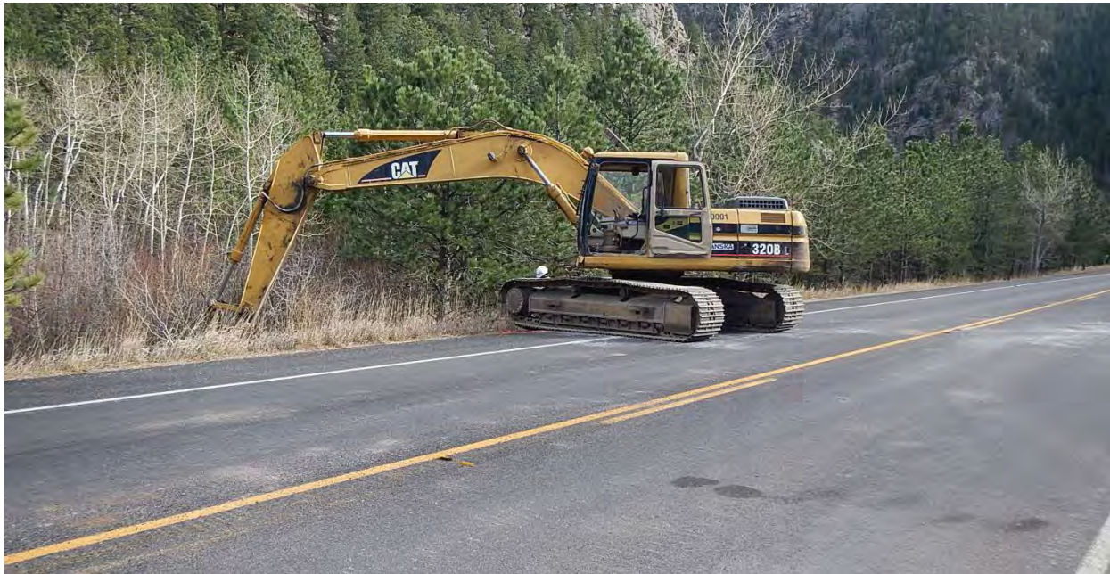
Figure 15 - MP 22, Emergency repair.
