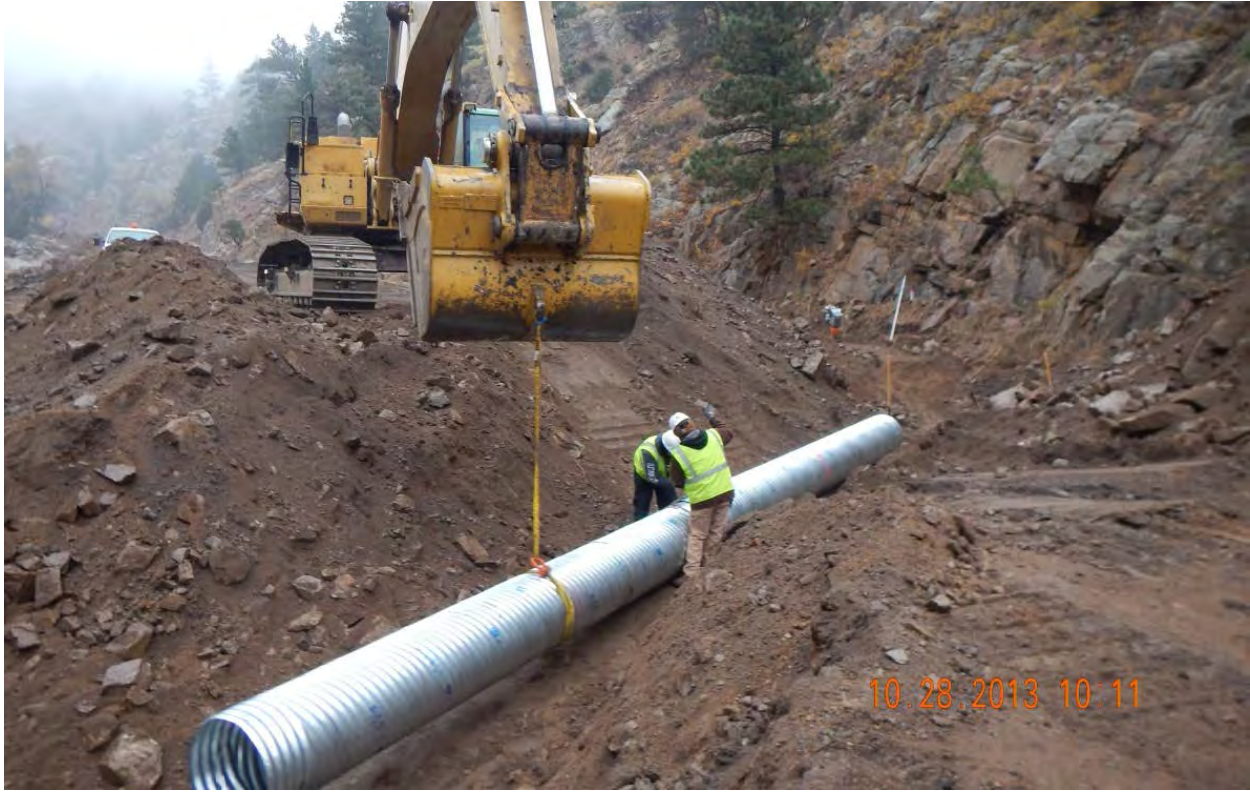
Figure 55 - MP 26.5, CMP repair.
