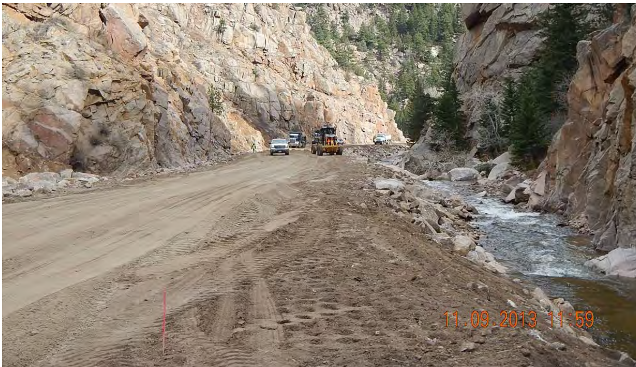
Figure 56 - MP 26.9, Facing northeast, Roadway repair.
