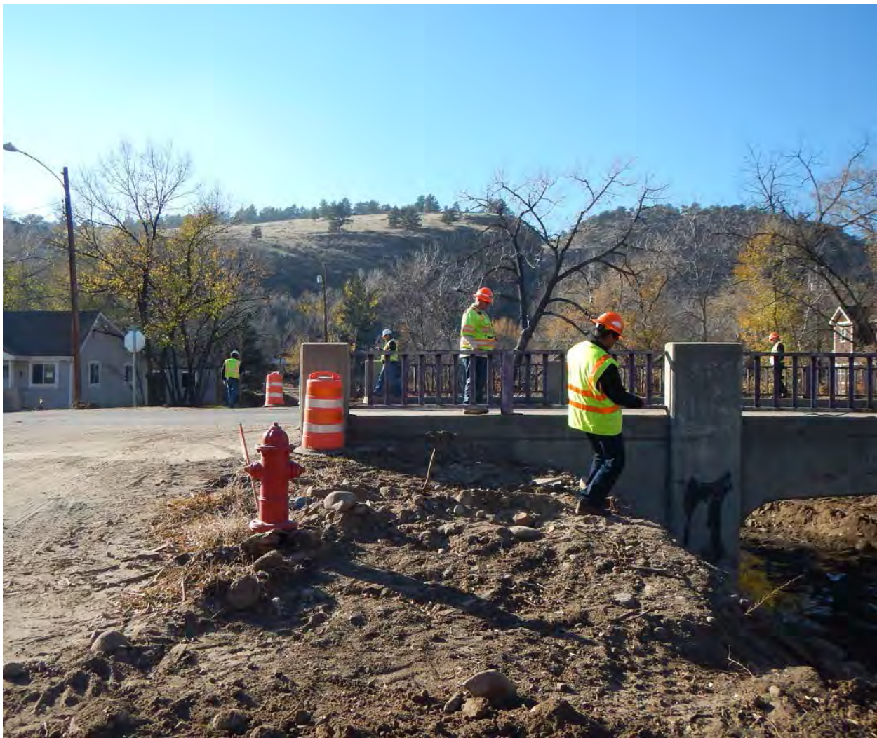
Figure 78 - MP 32.98, Facing west, Structure D-15-A embankment repair.
