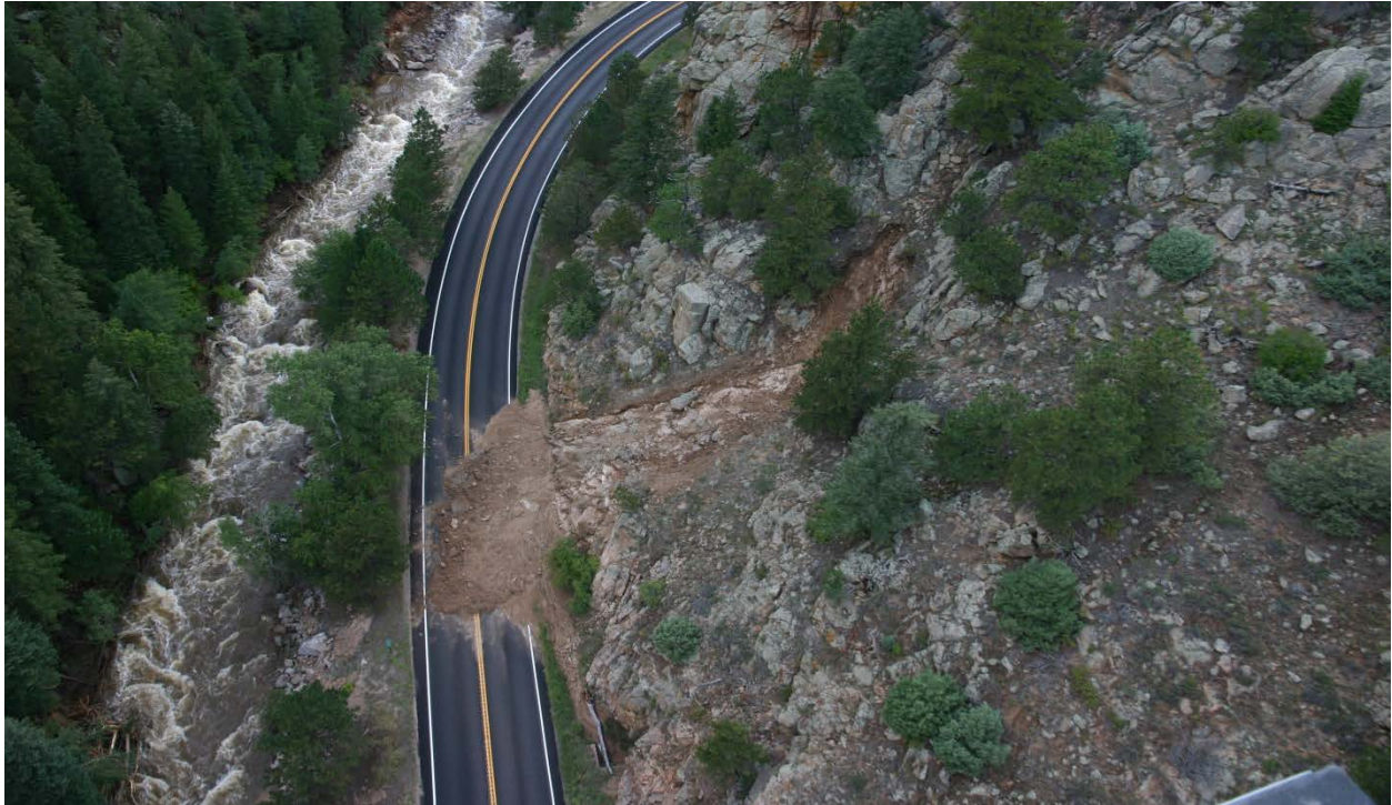
Figure 26 - MP 24.0, Rock slide covering both roadway lanes.
