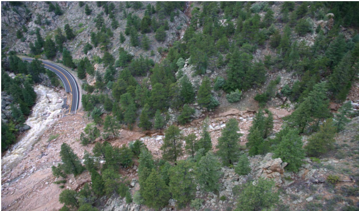
Figure 29 - MP 24.75, Rock slide covering roadway lanes. Embankment and roadway washout.
