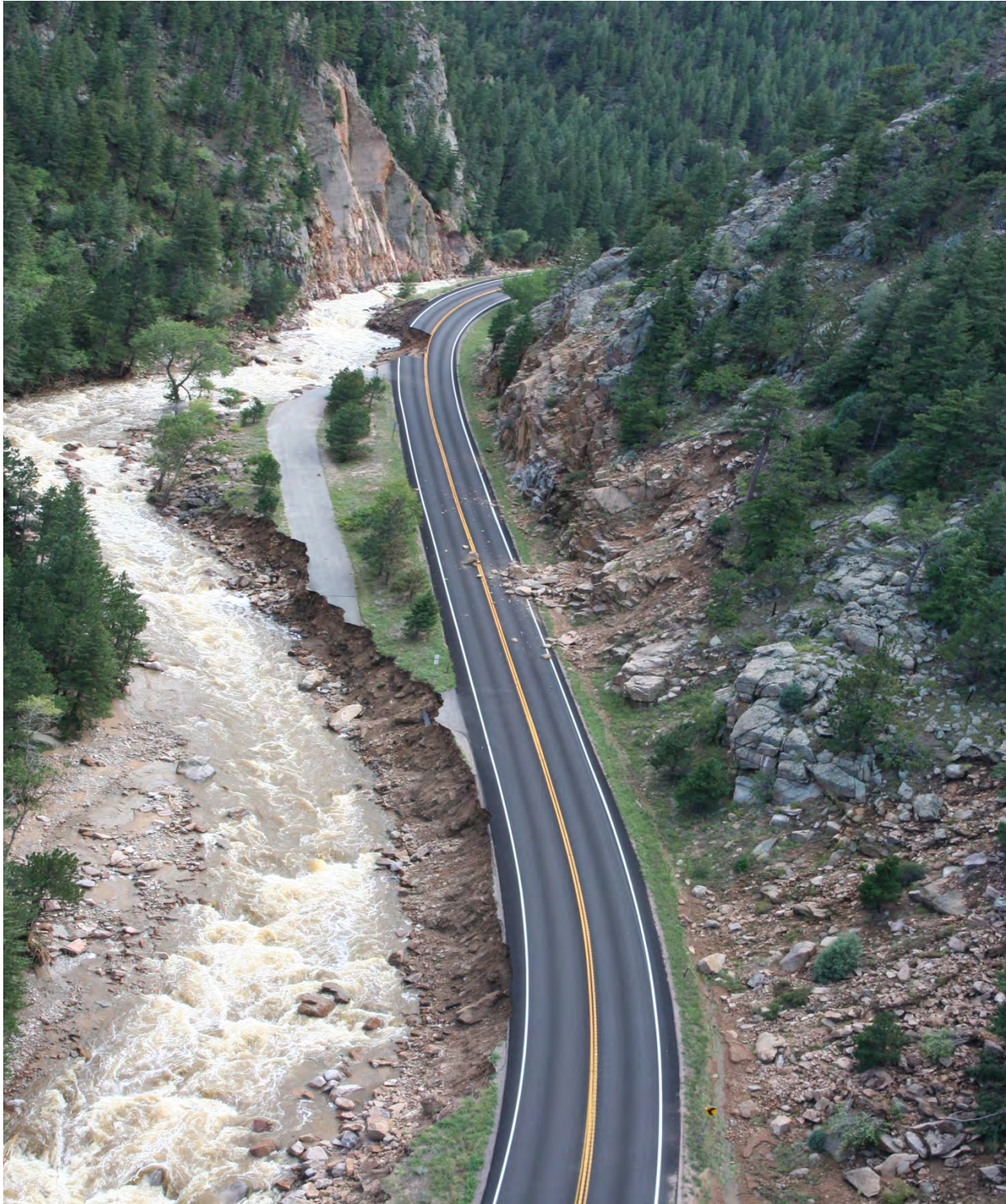
Figure 32 - MP 25.8, Embankment/pavement washout and rockslide.
