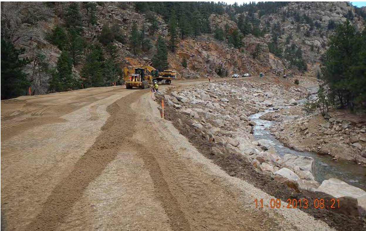
Figure 58 - MP 27.2, Facing north, Roadway repair.
