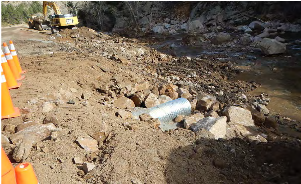
Figure 54 - MP 26.2, CMP Repair.
