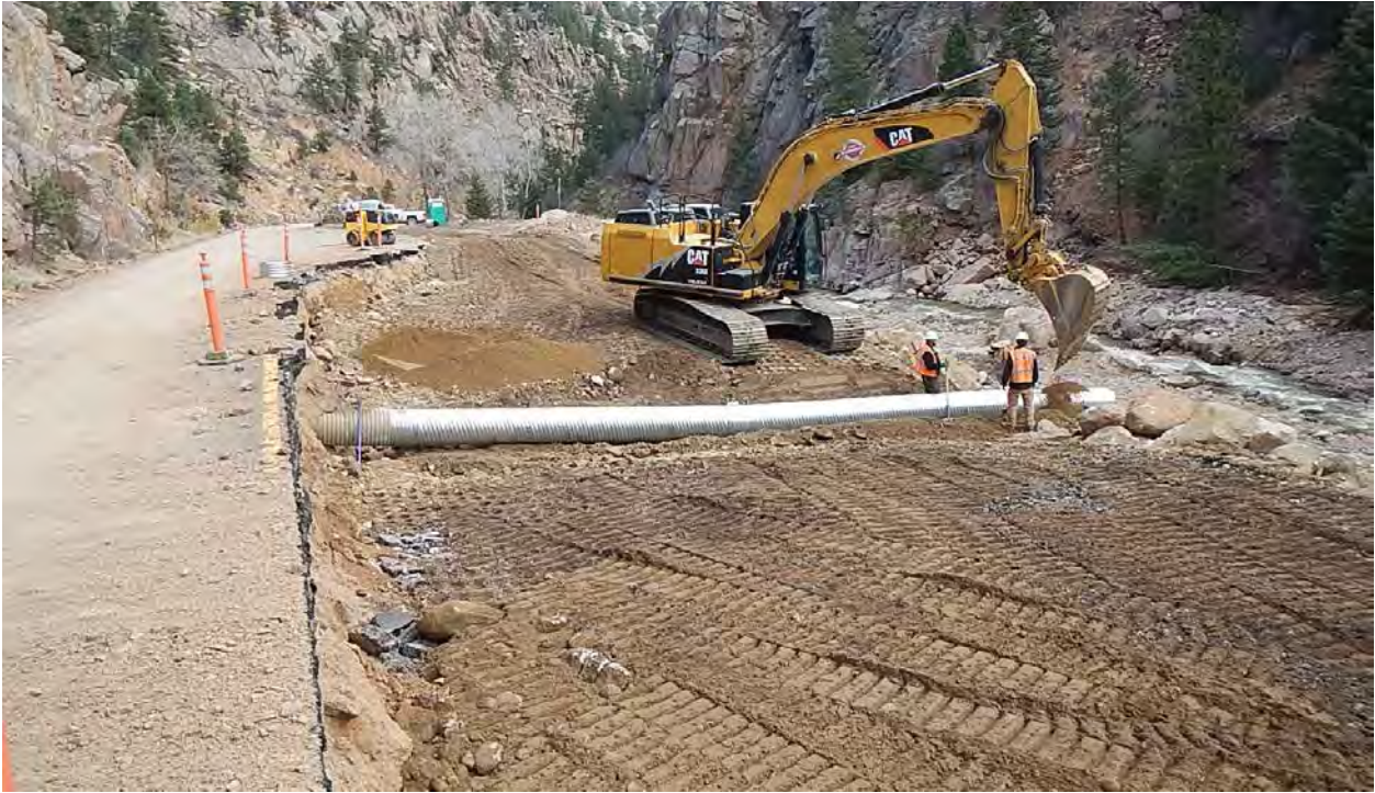
Figure 59 - MP 27.35, Facing North, Roadway and CMP repair.
