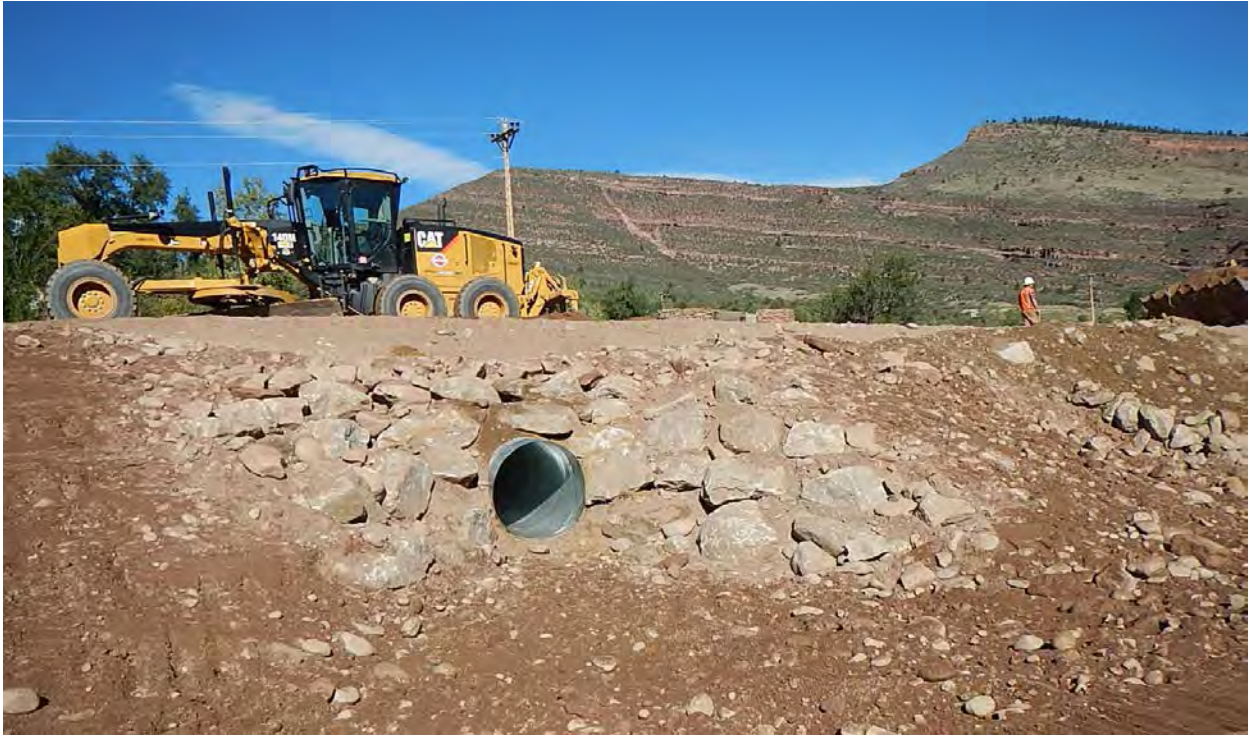
Figure 72 - MP 31.2, ER CMP installation complete.
