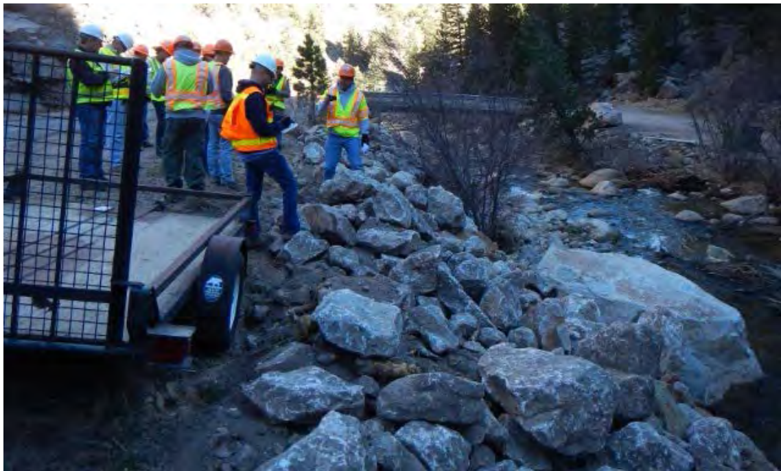
Figure 20 - MP 22.49, Eastbound roadway embankment repair.
