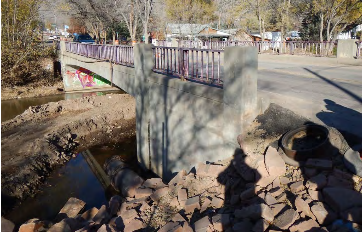
Figure 79 - MP 32.98, Facing northeast, Structure D-15-A temporary access.
