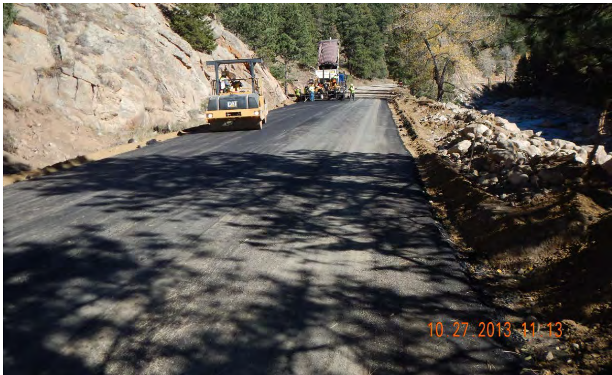
Figure 50 - MP 25.3 Facing east, Roadway repair.
