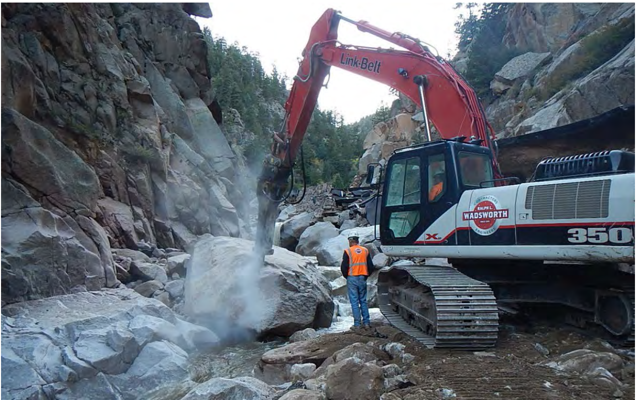
Figure 60 - MP 27.4, Looking South.
