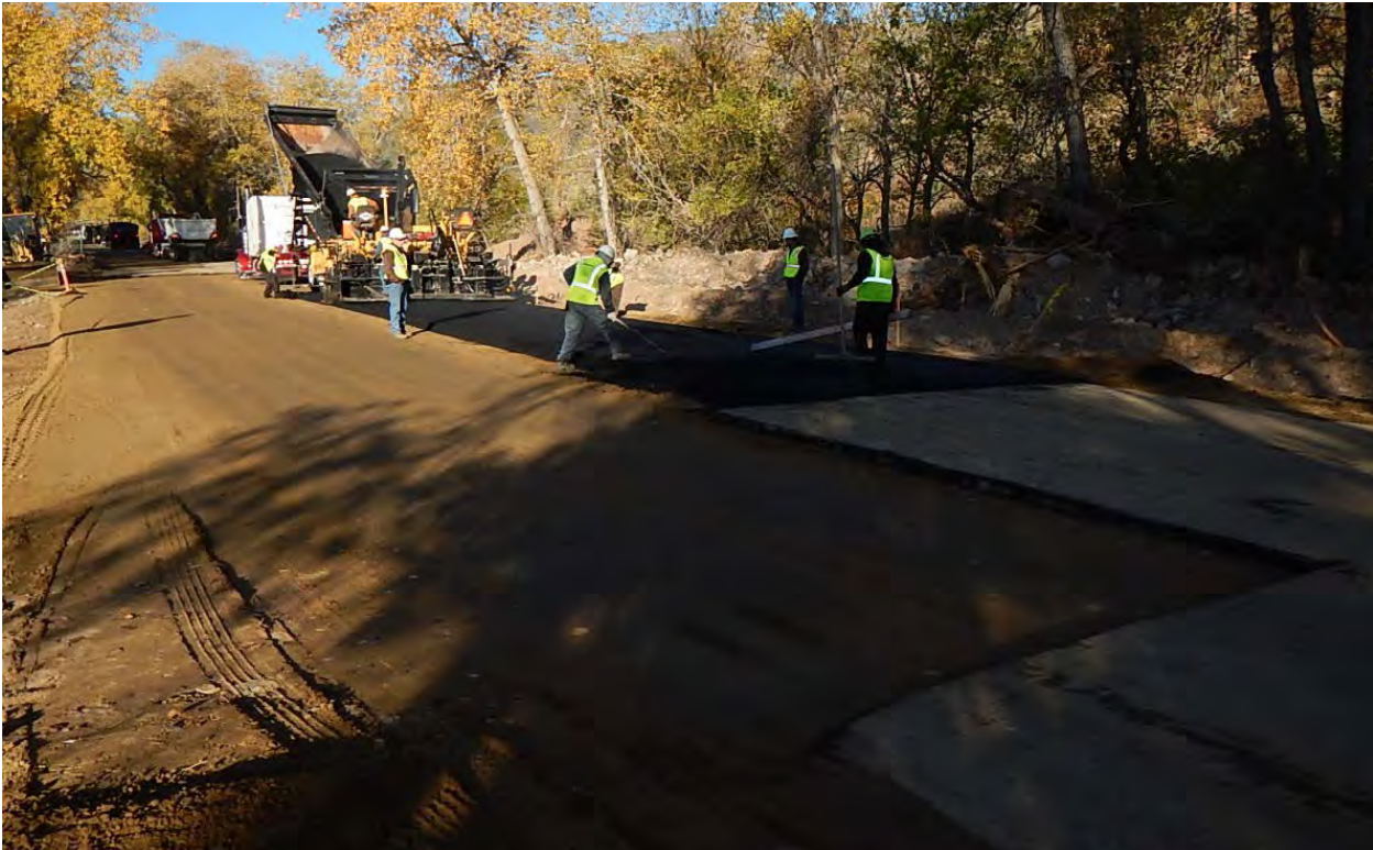
Figure 73 - MP 31.7, ER Paving operations.
