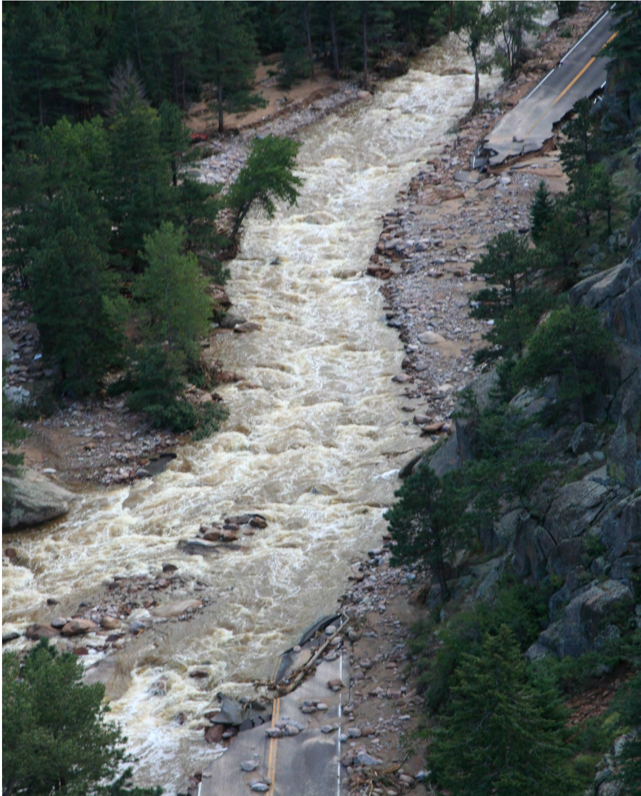
Figure 41 - MP 28.5, Complete wash out of the roadway due to lateral scour and overtopping of the roadway.
