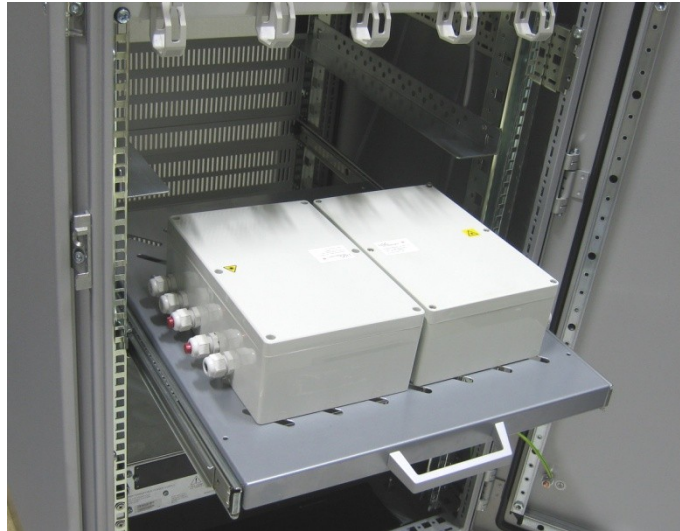
Figure 33: Mounting of splice boxes inside a rack
