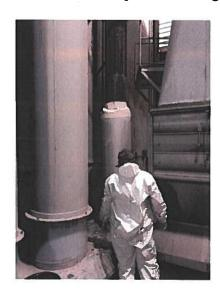
3. Emergency generator flue insulation enclosed behind metal cover and subsequently sealed at the top.
