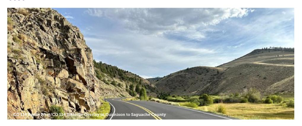
Crews completed resurfacing, leveling, widening shoulders and upgrading guardrails along 22 miles of Colorado Highway 114 in Gunnison and Saguache counties.
