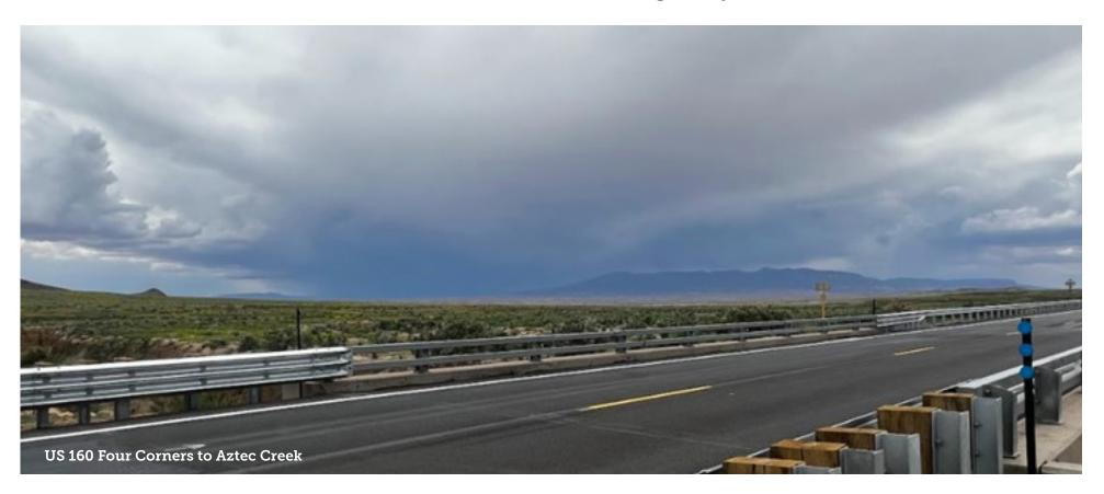
In June of 2023, US Highway 160 was successfully resurfaced from the Four Corners to Aztec Creek. The 9-mile stretch of highway included a full-depth reclamation and reconstruction.
