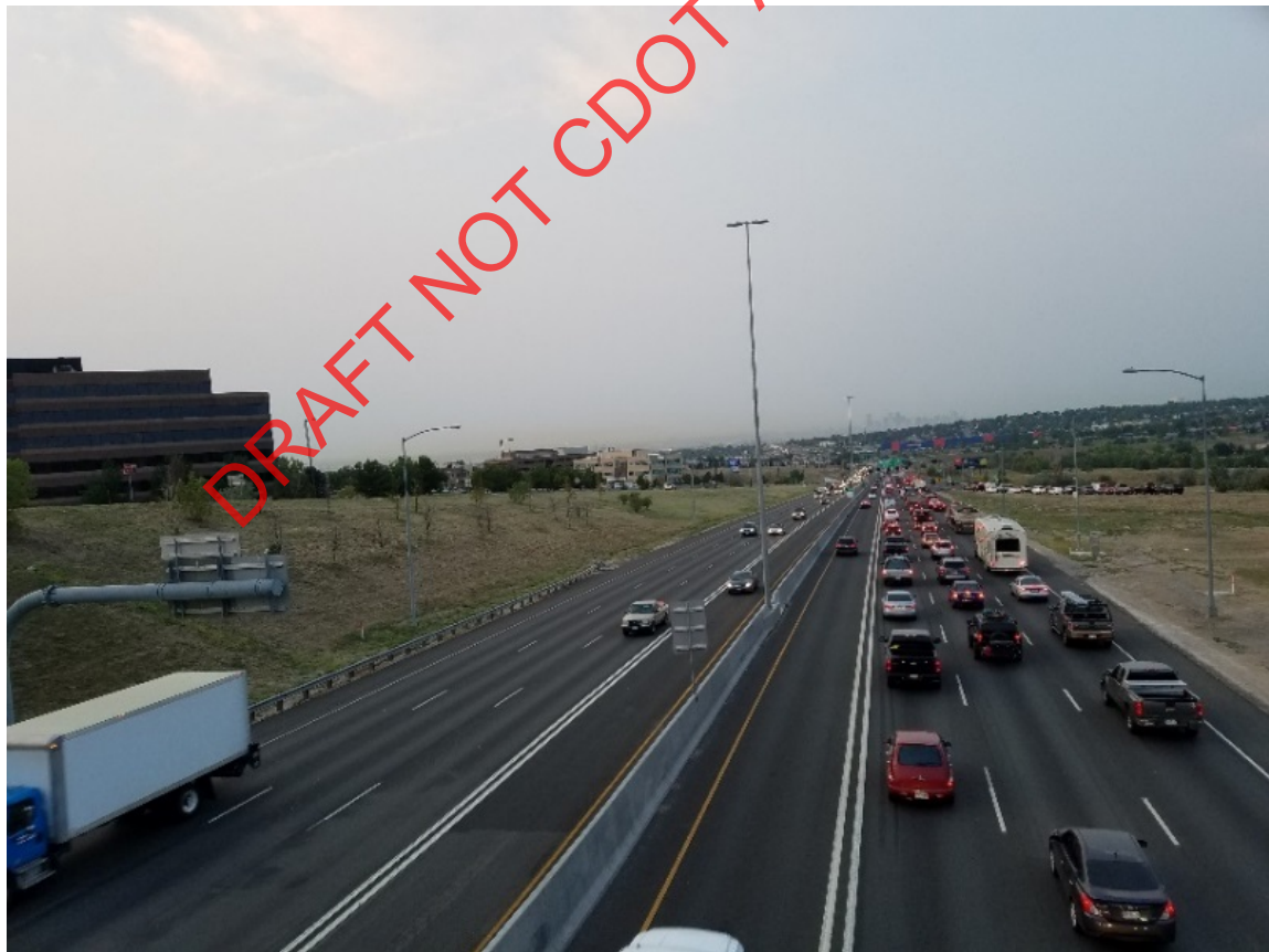
Figure 10 - On Thornton Pkwy overpass looking south (9/7/17 at 6:45am)
