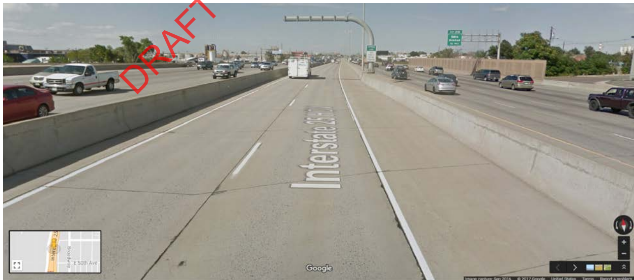
Figure 6 - Example Street View of I-25 HOV/Toll Lanes near 50th Avenue (Metro)
