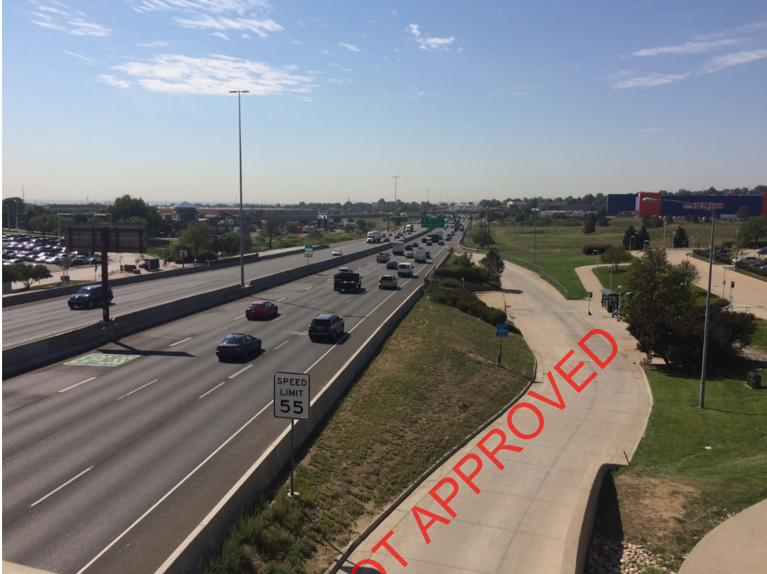
Figure 32 - RTD station on west side of I-25 just south of 88th Ave
