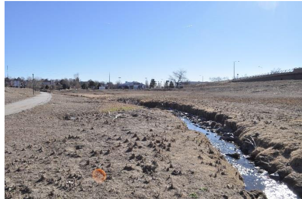
Photo 2: February 14, 2017 - Southernmost extent of Niver Creek within the project area.
