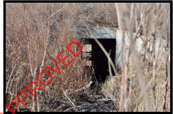
Figure 9. Niver Creek Tributary L Concrete Box Culvert
