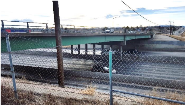
Photo 18. 88 th Avenue Bridge (5AM.3786)
