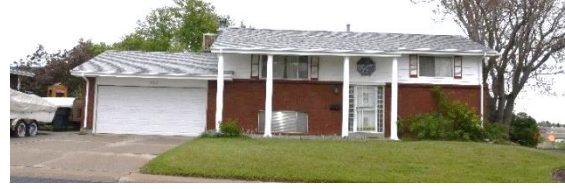
Photo 6. 5AM.3778, Bi-Level House
