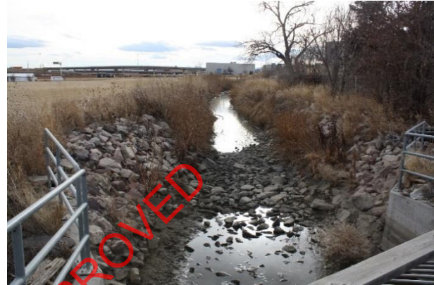
Photo 4. Colorado Agricultural Canal Segment (5AM.81 - Segment 5AM.81.1)
