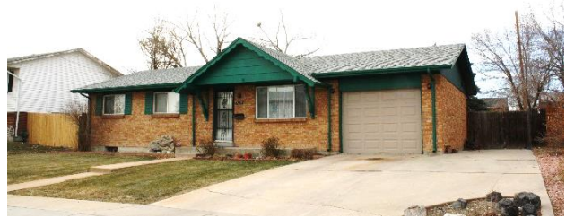
Photo 11. 5AM.3780, Ranch House
