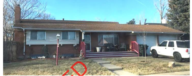
Photo 10. 5AM.3779, Rectangular Ranch House
