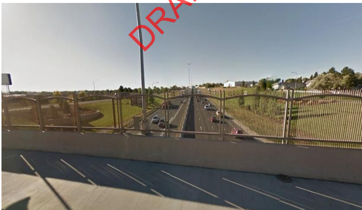
View south of I-25 from 84 th Street bridge
