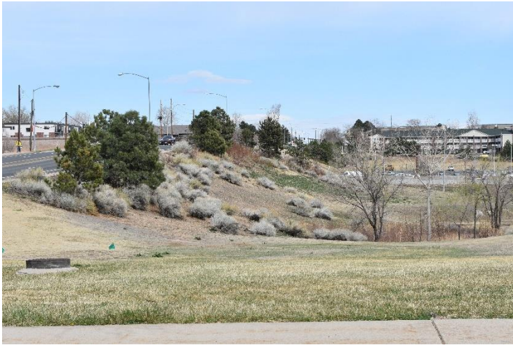
88 th Street Bridge Landscaping • View east of I-25 and 88 th Avenue bridge landscaping adjacent to RTD bus facility
