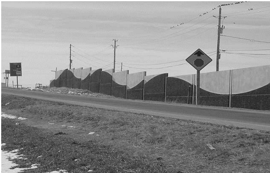
Figure 16-4 Combination Barrier: I-25 at Exit 188
