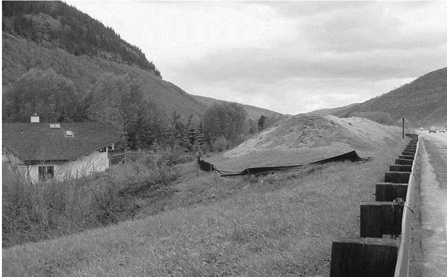
Figure 16-4 Combination Barrier: I-25 at Exit 188
