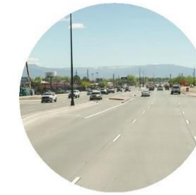
Suburban Places: Ground Level
