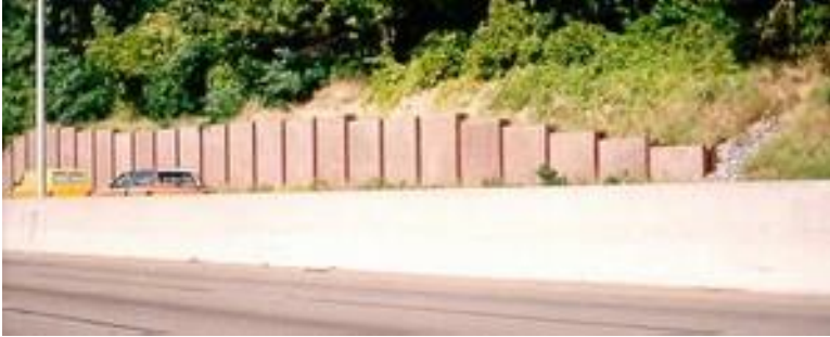
Figure 16.9. Barrier End Treatment: Buried Into Existing Ground
