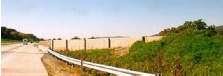
Figure 16-8 Barrier End Treatment: Stepped Panel
