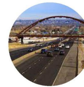
Freeway: Overpass Level
