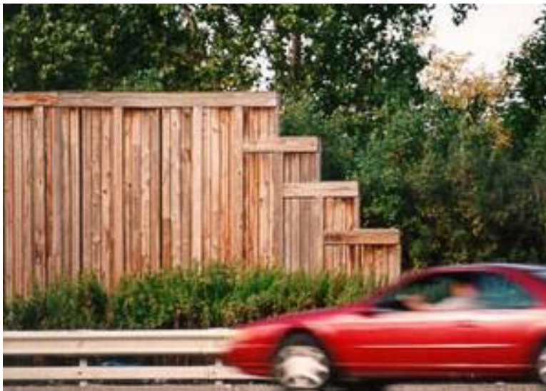
Figure 16-8 Barrier End Treatment: Stepped Panel
