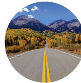
Rural Mountain Road: Ground Level
