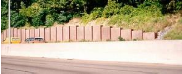
Figure 16.9. Barrier End Treatment: Buried Into Existing Ground
