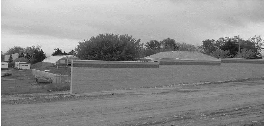
Figure 16-2 Post-and-Panel Noise Barrier Mounted on Type 7 Barrier: US-6 in Lakewood
