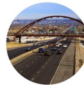
Freeway: Overpass Level
