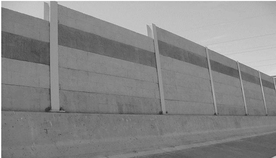
Figure 16-2 Post-and-Panel Noise Barrier Mounted on Type 7 Barrier: US-6 in Lakewood
