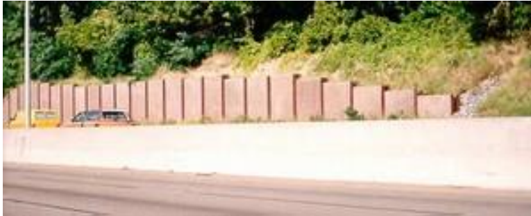
Figure 16.9. Barrier End Treatment: Buried Into Existing Ground
