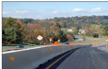
JJ Hooks Concrete Barrier
