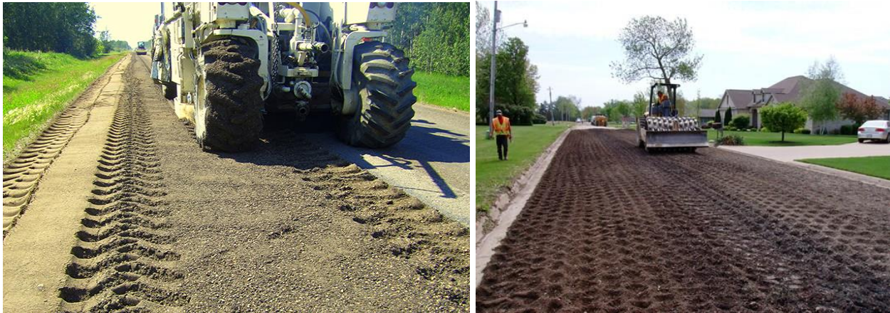
Figure 5.9 Photos of Full Depth Asphalt Reclaimed Base
