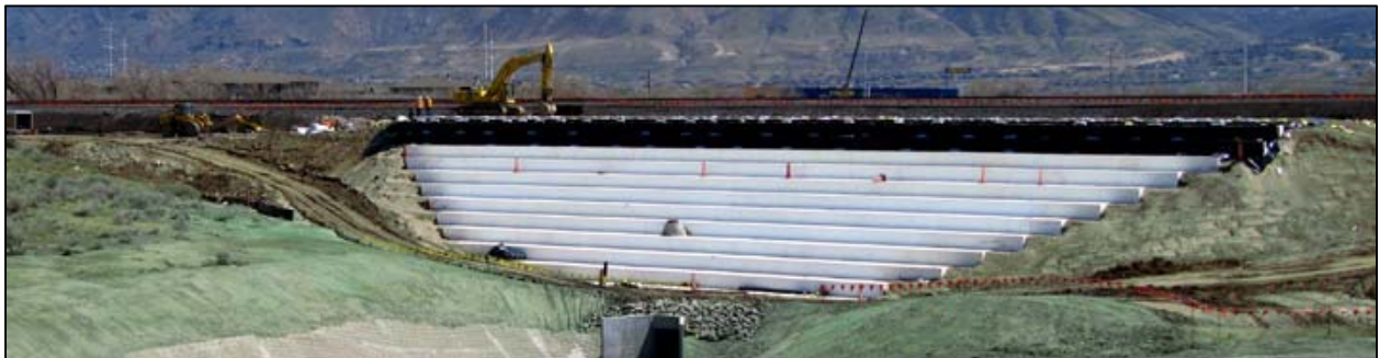
Photograph 15: Light-weight EPS foam blocks being used to bridge over soft clay deposits for new embankment construction.
