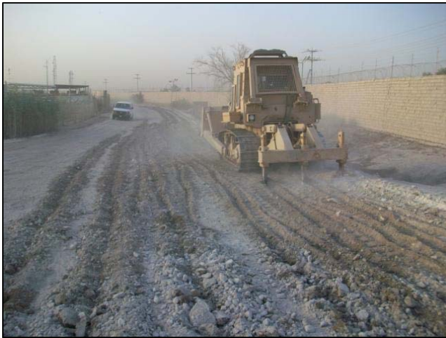
Photographs 2 and 3: Foundation preparation by means of using a dozer with a ripper attachment or a tractor with a disk to open the subgrade soils.
