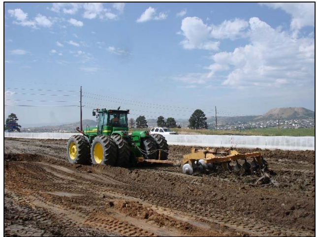
Photographs 2 and 3: Foundation preparation by means of using a dozer with a ripper attachment or a tractor with a disk to open the subgrade soils.
