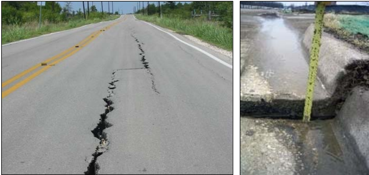
Photographs 17 and 18: Damage to asphalt pavement and separation along a concrete construction joint as a result of swelling soils.
