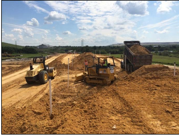
Photographs 13 and 14: Accelerated consolidation being achieved through the use of surcharging and wick drains.
