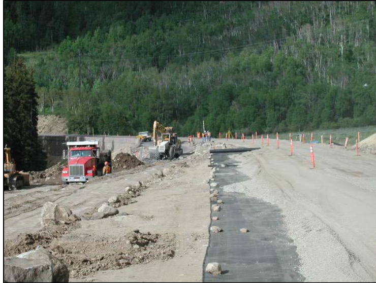
Photograph 22: Geotextile installation over soft, unstable subgrade soils.
