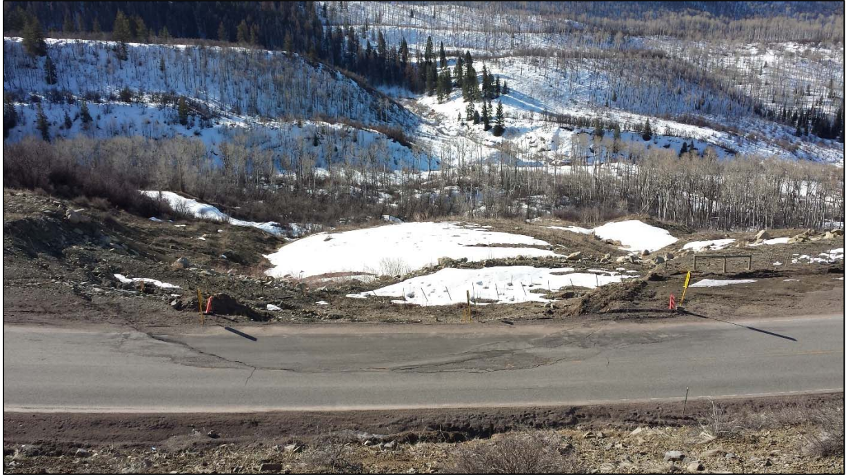
Photograph 16: Landslide that developed as a result of embankment construction over a weak clay deposit.
