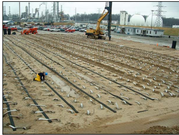
Photographs 13 and 14: Accelerated consolidation being achieved through the use of surcharging and wick drains.
