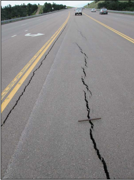
Photographs 11 and 12: Resultant pavement damage due to differential settlement caused by consolidation of saturated clays beneath a high embankment.
