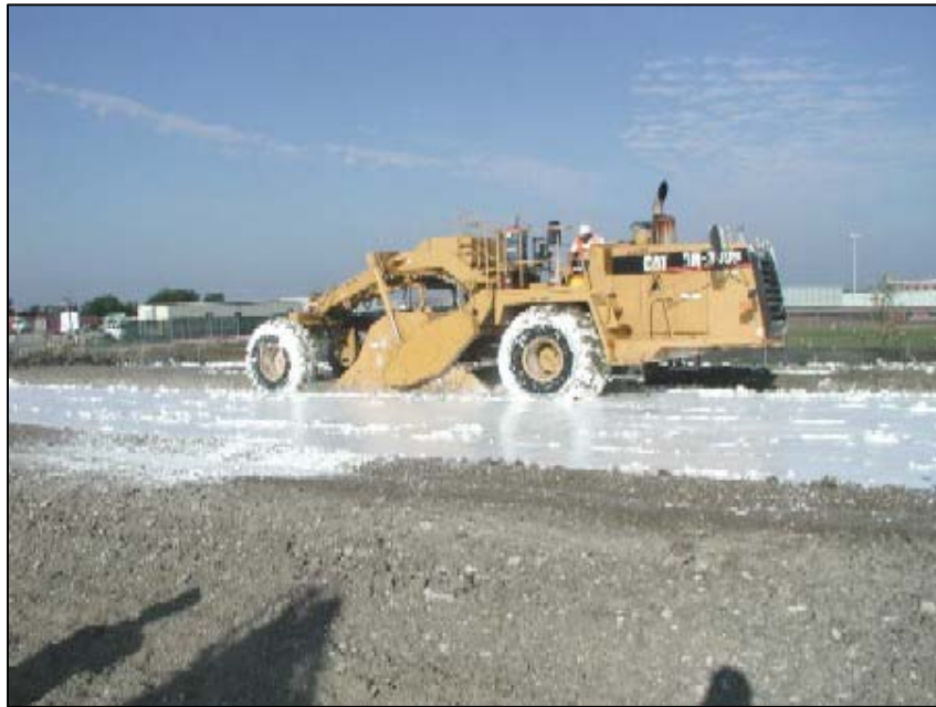
Photograph 19: Mixing a lime slurry into subgrade soils to reduce the swell potential.
