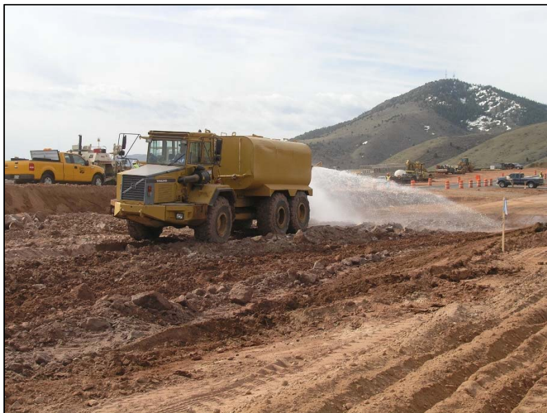
Photograph 6: Water truck being used to moisture condition soils in preparation for compaction.
