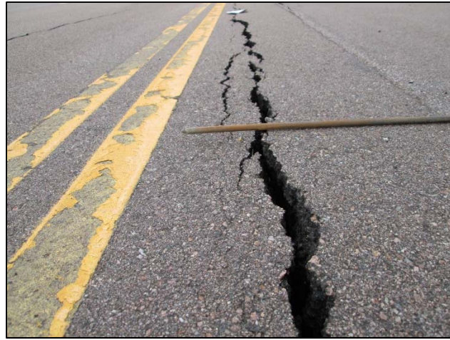
Photographs 11 and 12: Resultant pavement damage due to differential settlement caused by consolidation of saturated clays beneath a high embankment.
