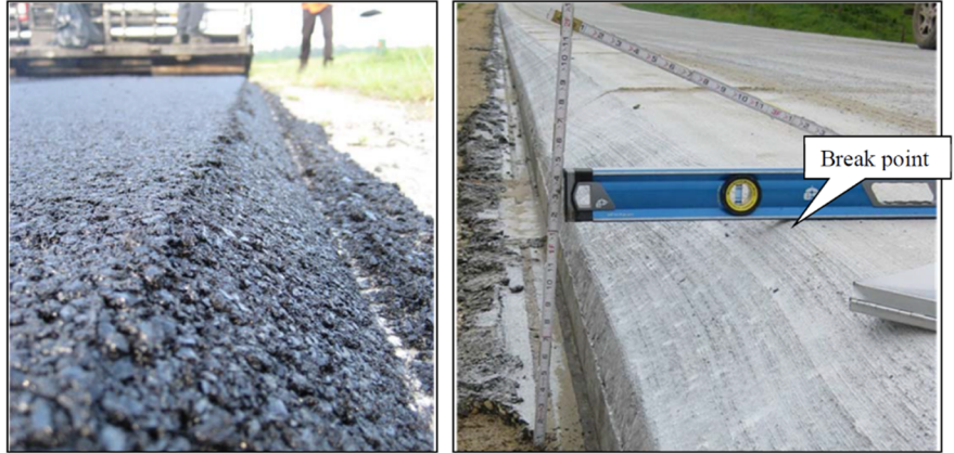
Figure 1. Safety Edge placed on AC and PCC
