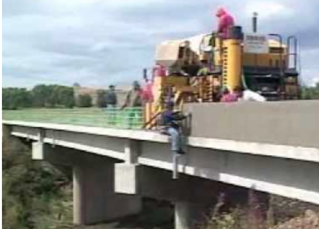
Figure 3: Slip Form Paver
