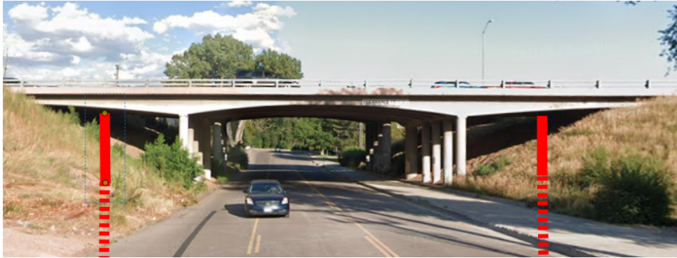
Figure 1: Existing I-25 Bridge Over Ellston
