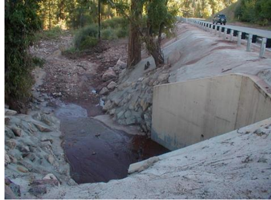
Photo 9.4 Culvert outlet
