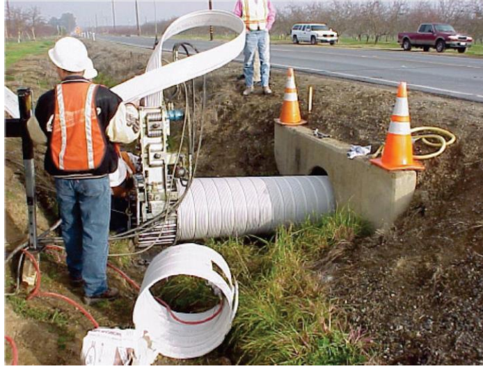
Photo 5 Spirally-wound pipe liner being installed
