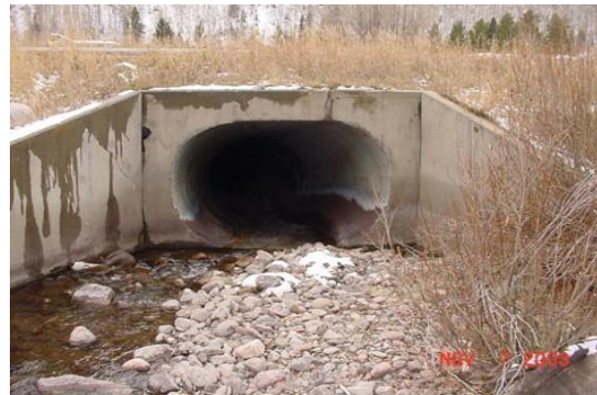
Photo 9.2 Same improved inlet after construction on Interstate Highway 70
