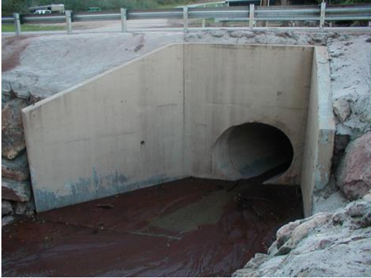
Photo 9.3 Culvert outlet
