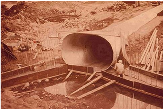
Photo 9.1 Improved inlet during construction on Interstate Highway 70
