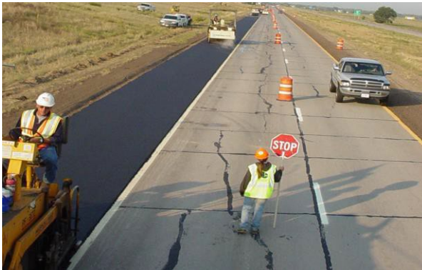
Region 4 Fort Morgan overlay project.
