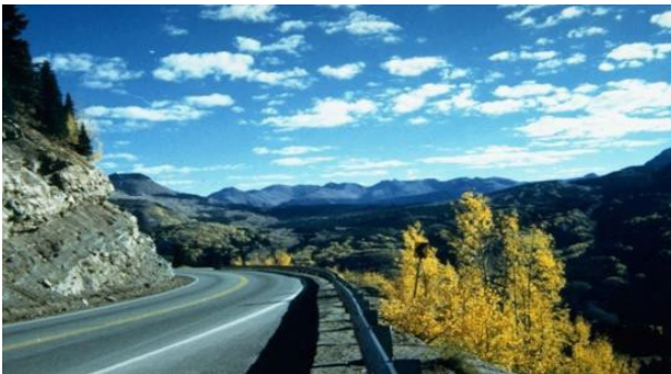
Region 5 Colorado's Famous "Million Dollar Highway" Part of the San Juan Scenic Skyway US 550
