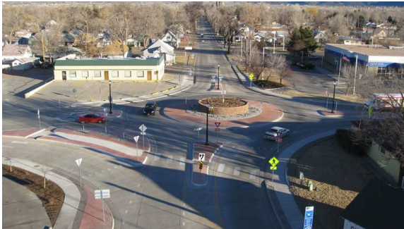
Region 2 Roundabout project in Canon City
