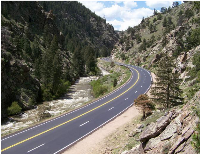
Region 1 U.S. Hwy. 6 Clear Creek Canyon: rock fall mitigation
