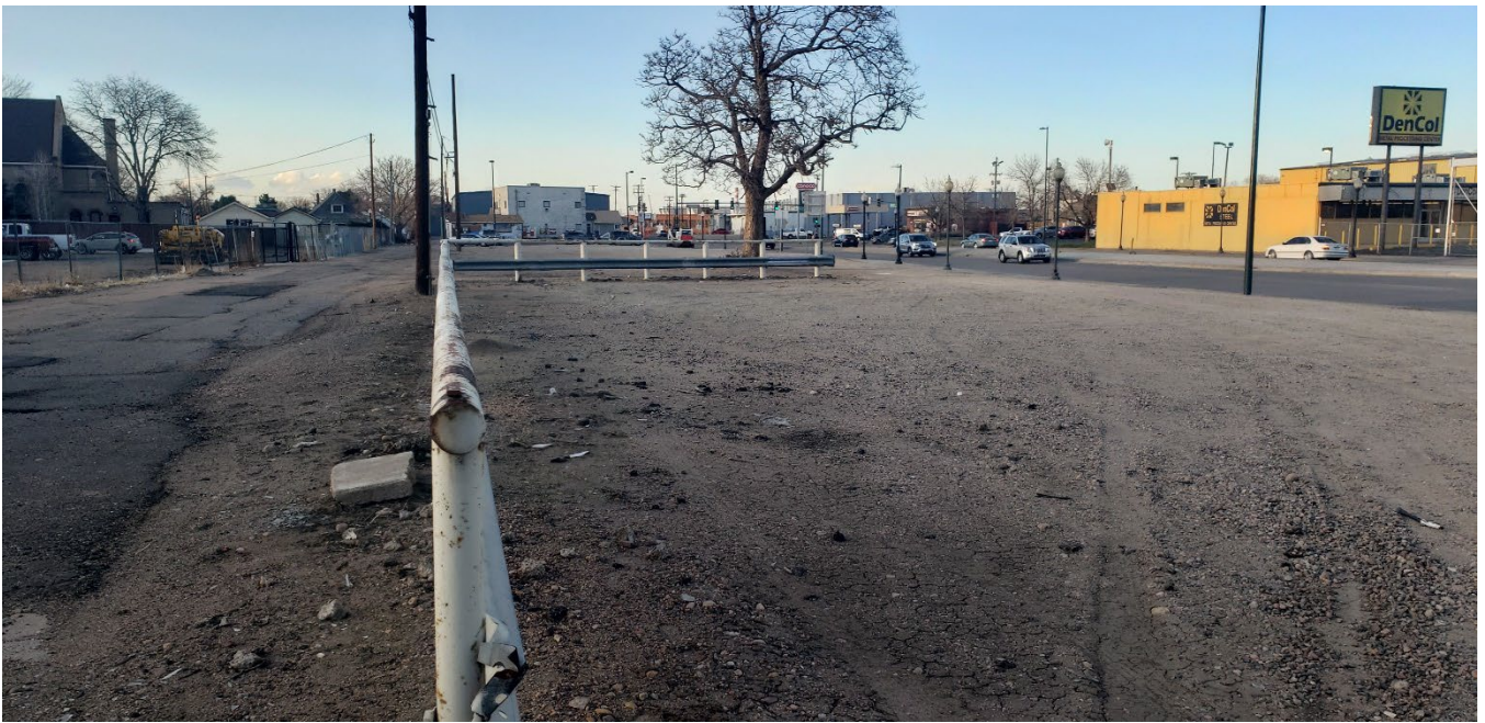
View of guard rail. Taken from the West, looking North
