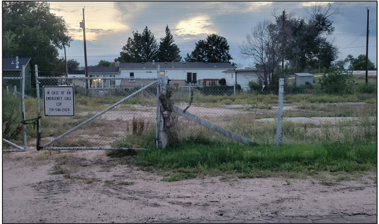
Subject view from the east on Golden Street, between 4 th and 5 th Street looking west.
