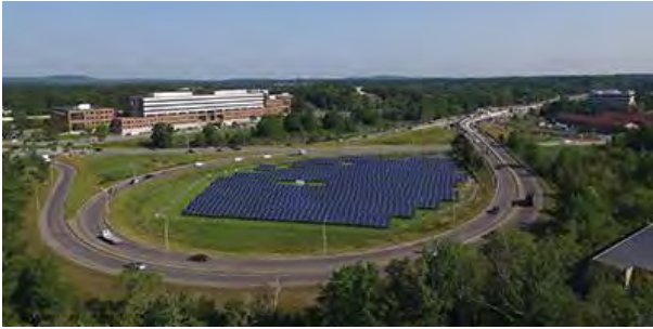
MassDOT-installed solar panels in the ROW at Exit 13 North on I-90 in Framingham, MA
