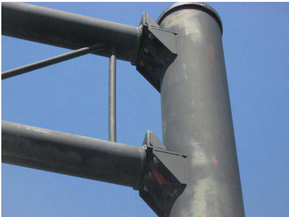
**Type 013:** Double arm truss, bolted connection on bearing plates
