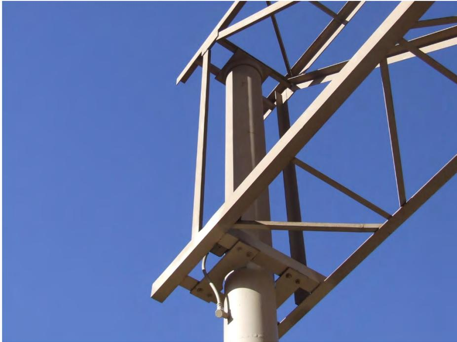
**Type 009:** Double arm (angle) truss, cap connection
