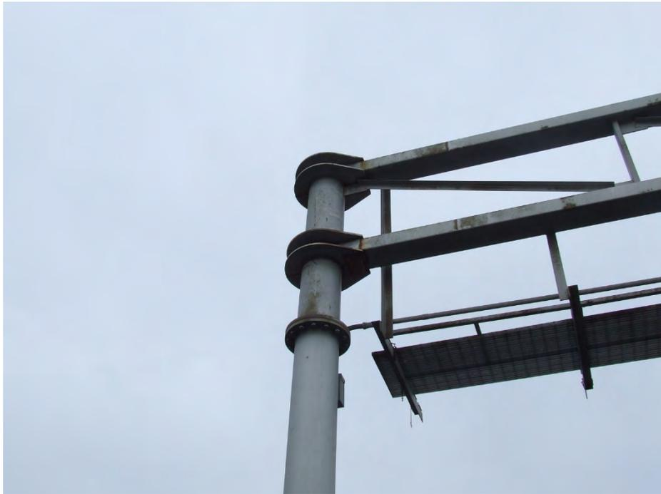
**Type 030:** Double arm, bracket welded to vertical, vertical bolted connection
