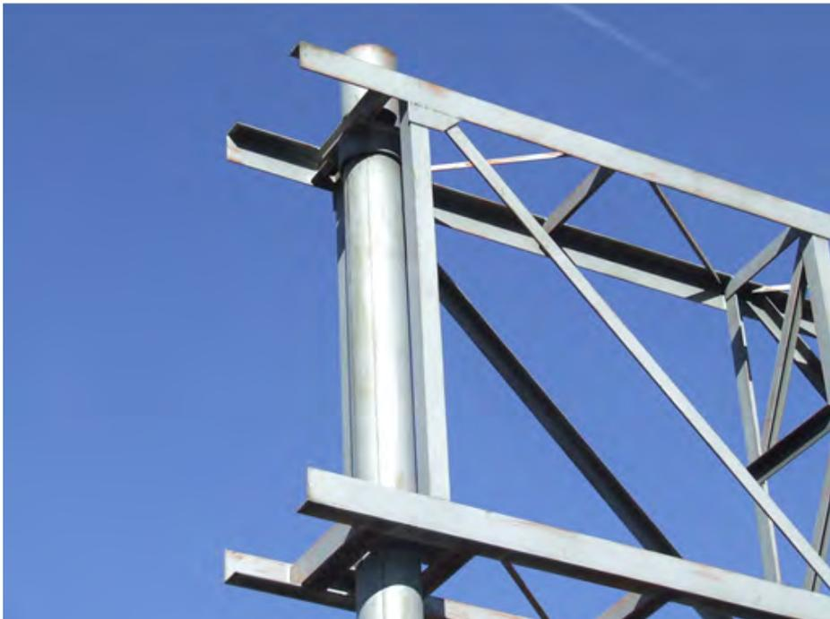
**Type 018:** Double arm box truss, collar connection
