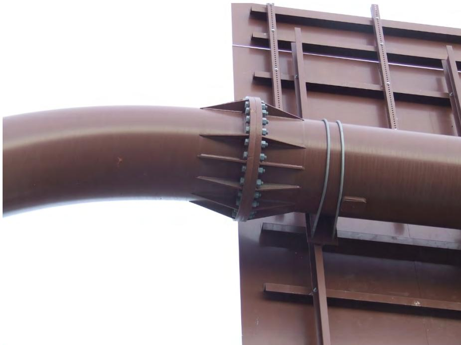
**Type 002:** Monotube, horizontal bolted connection, stiffened flanges
