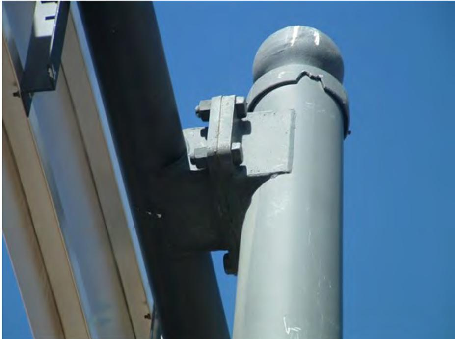
**Type 047:** Single arm, horizontal bolted connection to simplex plate on front of pole
