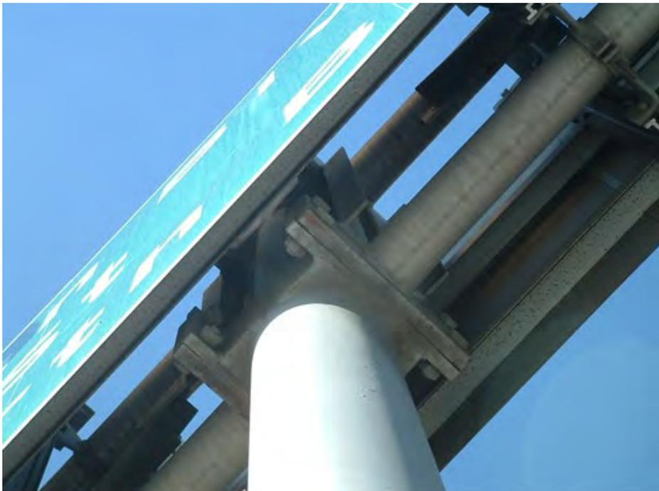
**Type 032:** Double face sign, double arm, double horizontal bolted connection to simplex plate
