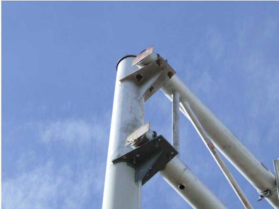
**Type 015:** Double arm truss, U-bolt fitted connection on bearing plates on front of pole
