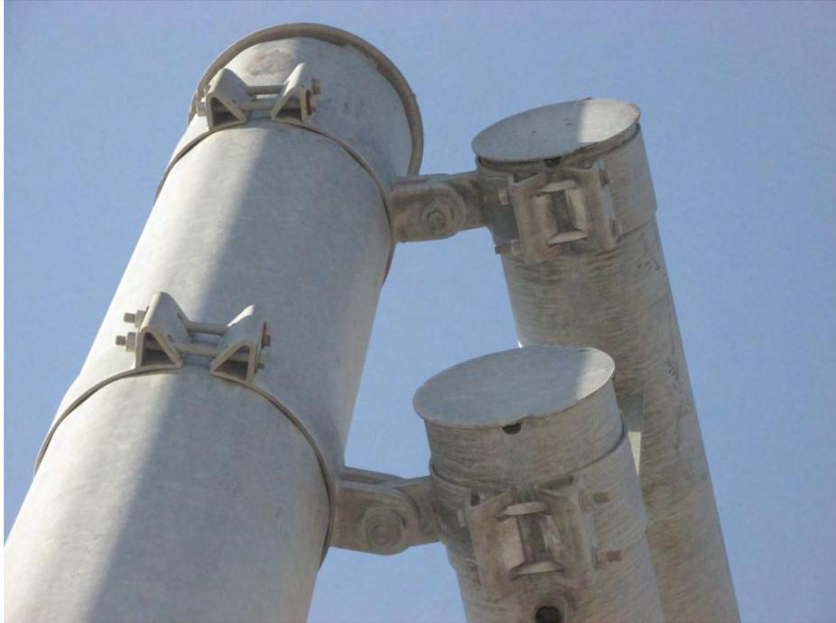
**Type 014:** Double arm, 3 finger collar connection, or 3 finger U-bolt clamp connection
