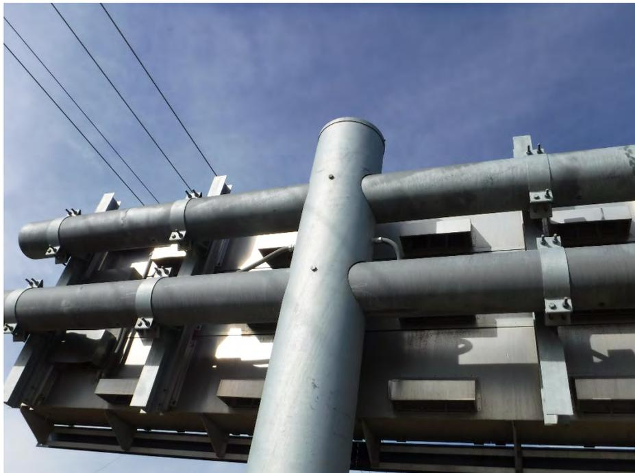
**Type 042:** Double arm, pipe fitted through vertical
