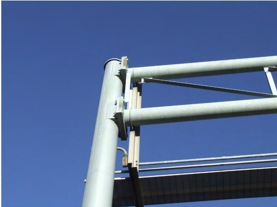
**Type 003:** Double arm, horizontal bolted connection to simplex plate
