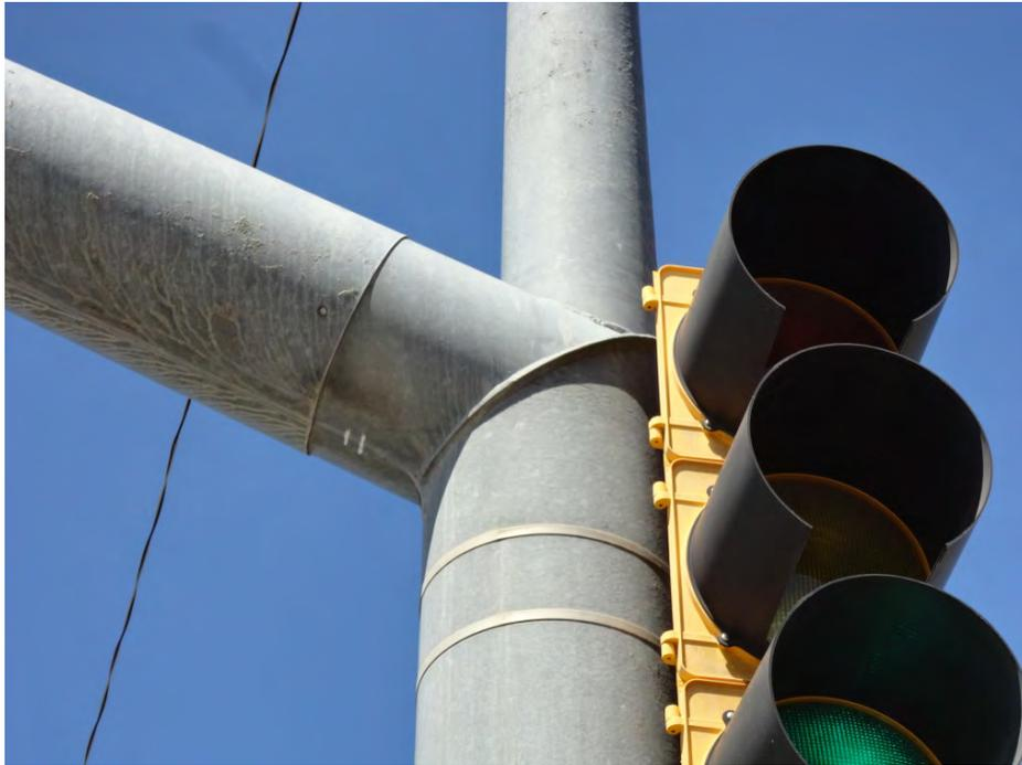
**Type 108:** Single arm, angled weld directly to column, with or without vertical pole on top
