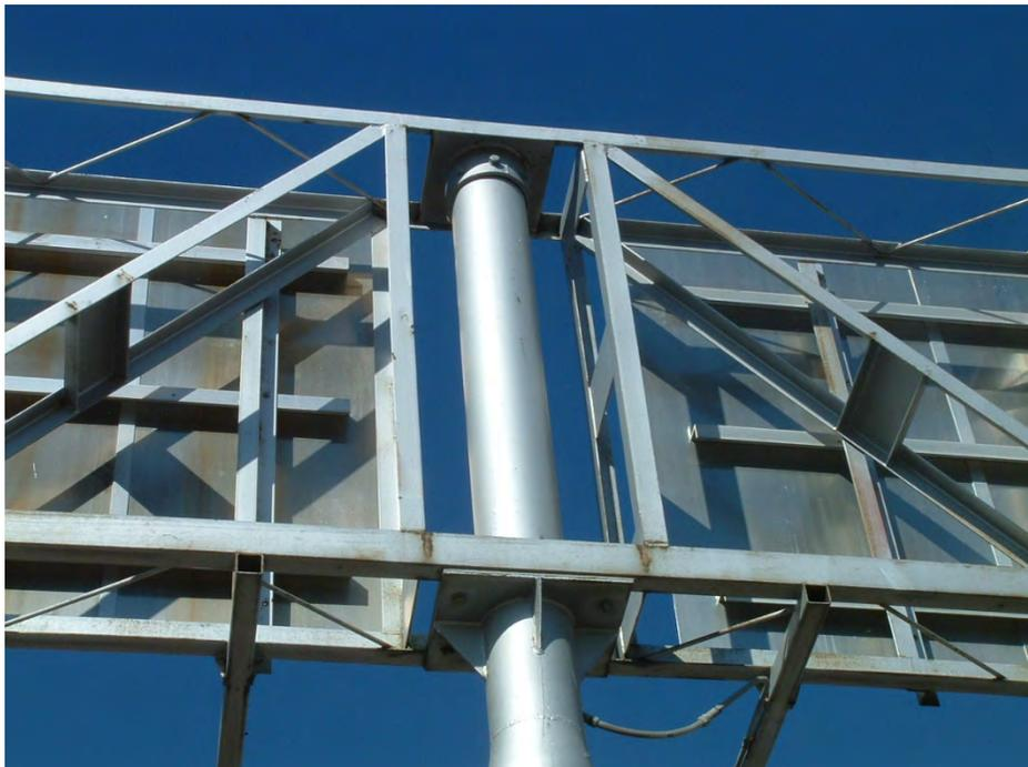
**Type 019:** Double arm box truss, cap connection
