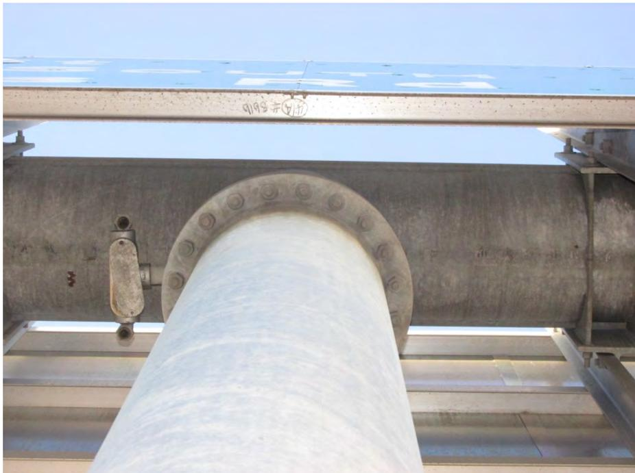
**Type 008:** Double face sign, single arm, cap-T horizontal bolted connection
