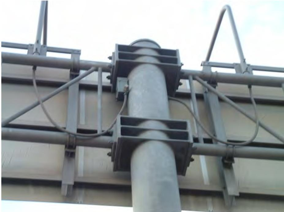
**Type 038:** Double arm, double horizontal bolted connection to simplex plate with welded stiffeners
