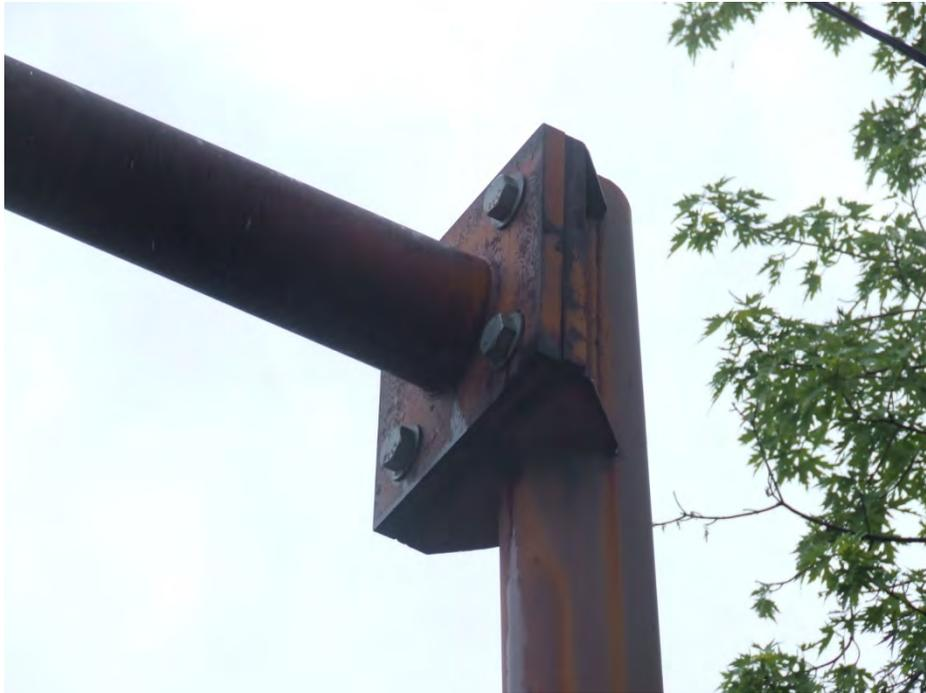
**Type 102:** Single arm, 4 bolt connection to simplex plate with welded stiffener
