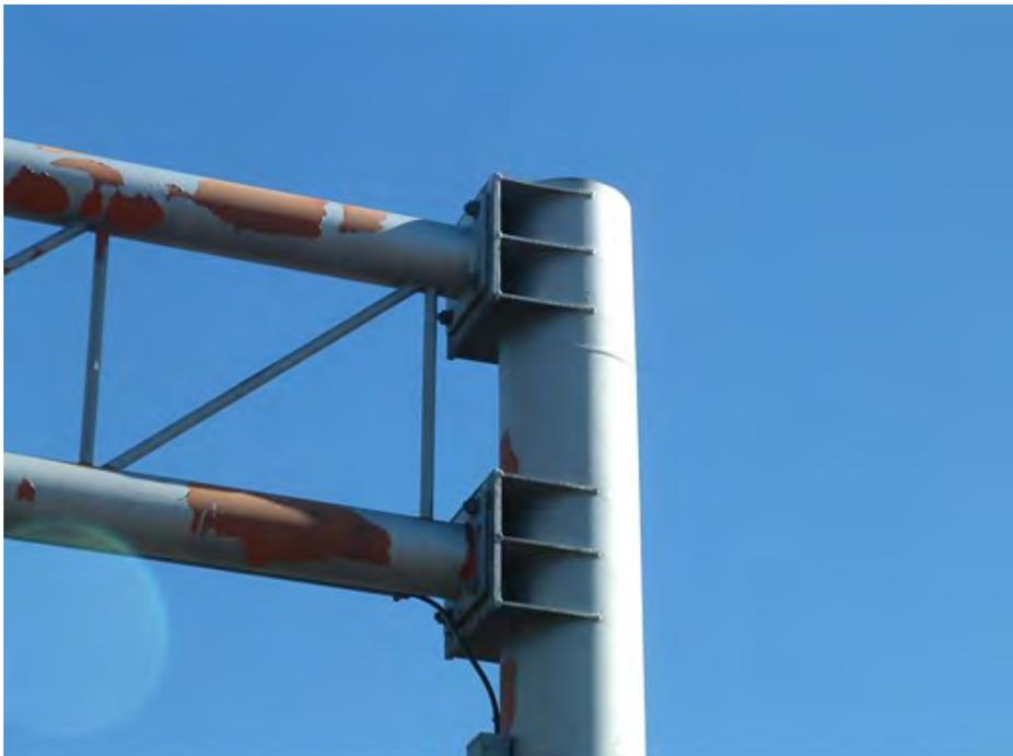
**Type 027:** Double arm frame, horizontal bolted connection to simplex plate with welded stiffener
