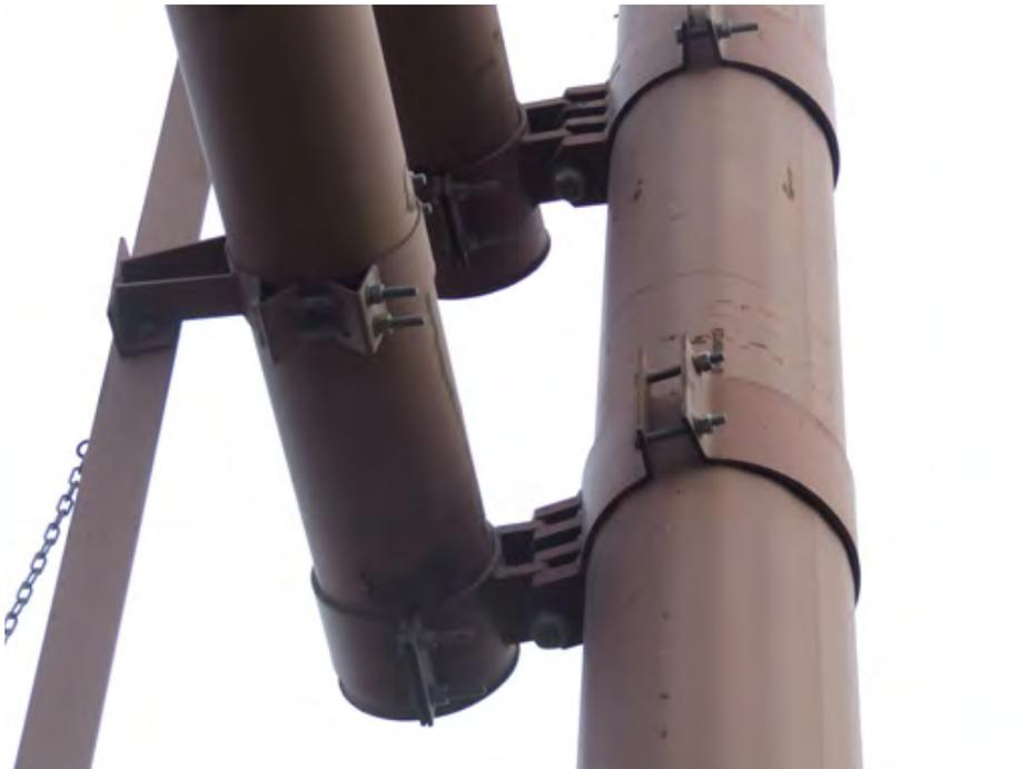
**Type 024:** Double arm, 6 finger collar connection, or 6 finger U-bolt clamp connection
