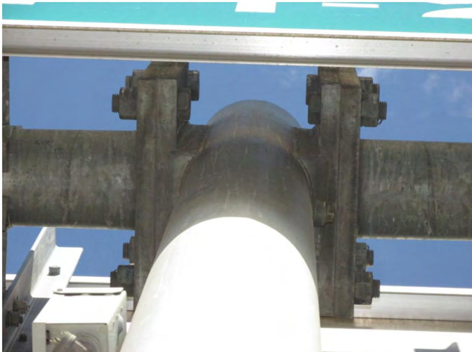
**Type 010:** Double face sign, single arm, double horizontal bolted connection to simplex plate
