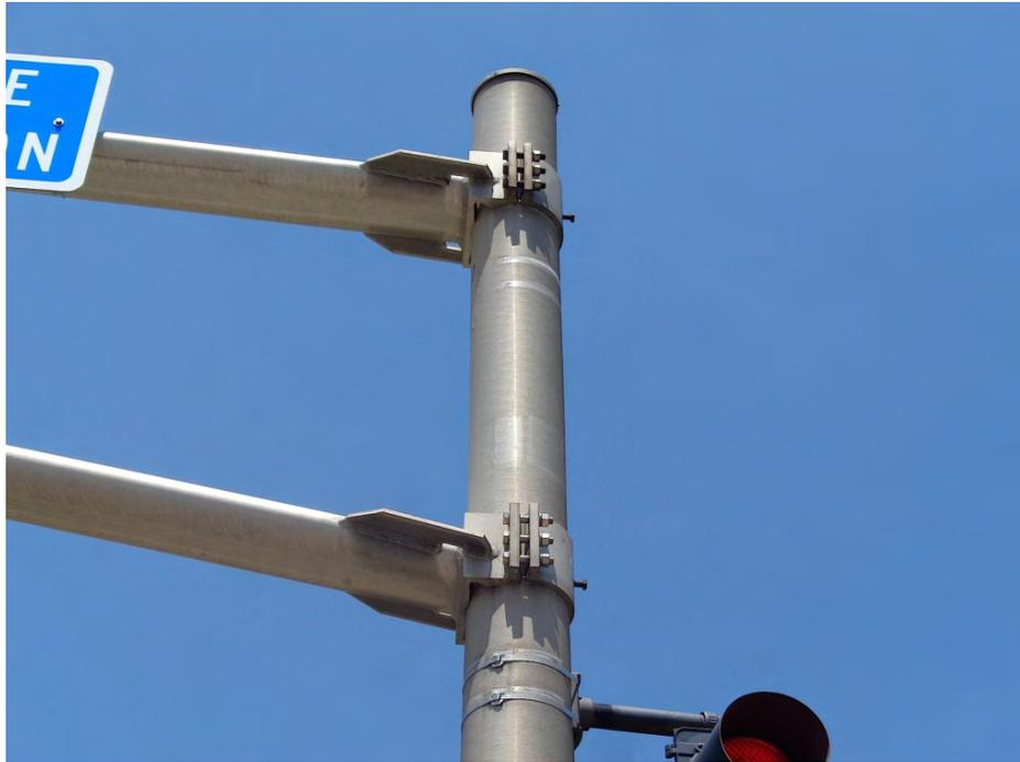
**Type 110:** Double arm, clamped connection
