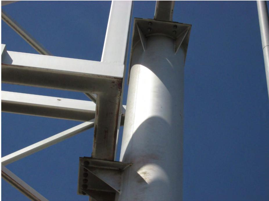
**Type 041:** Double arm box truss, bolted connection to top of pole and lower bearing plate
