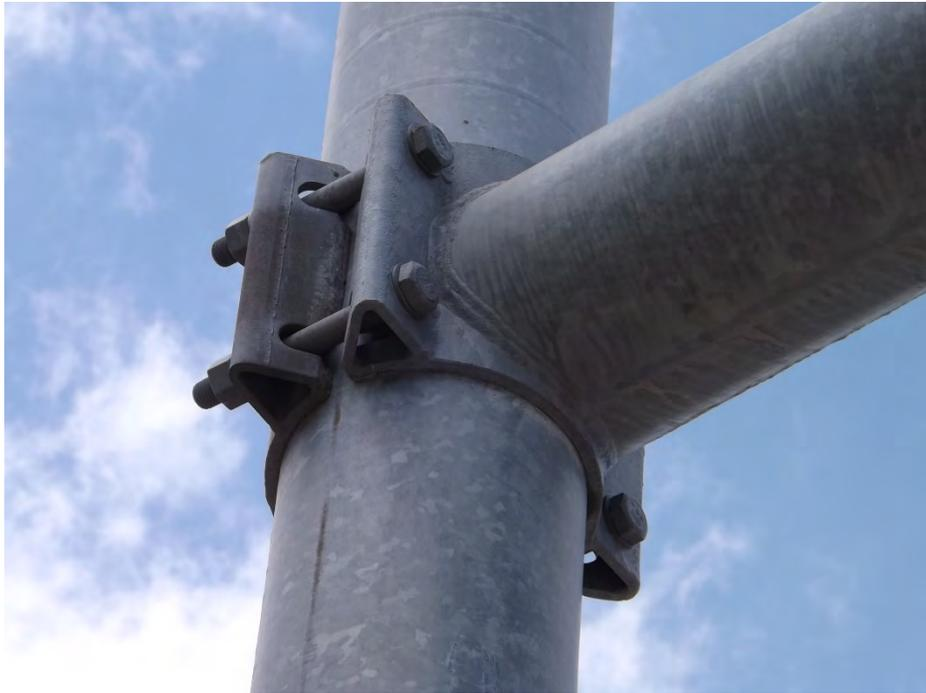
**Type 112:** Single arm, butterfly clamped connection
