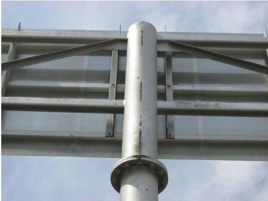
**Type 033:** Double arm, round column, vertical bolted cap connection
