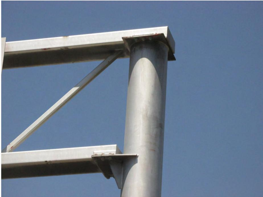
**Type 012:** Double arm truss, bolted connection to top of pole and lower bearing plate
