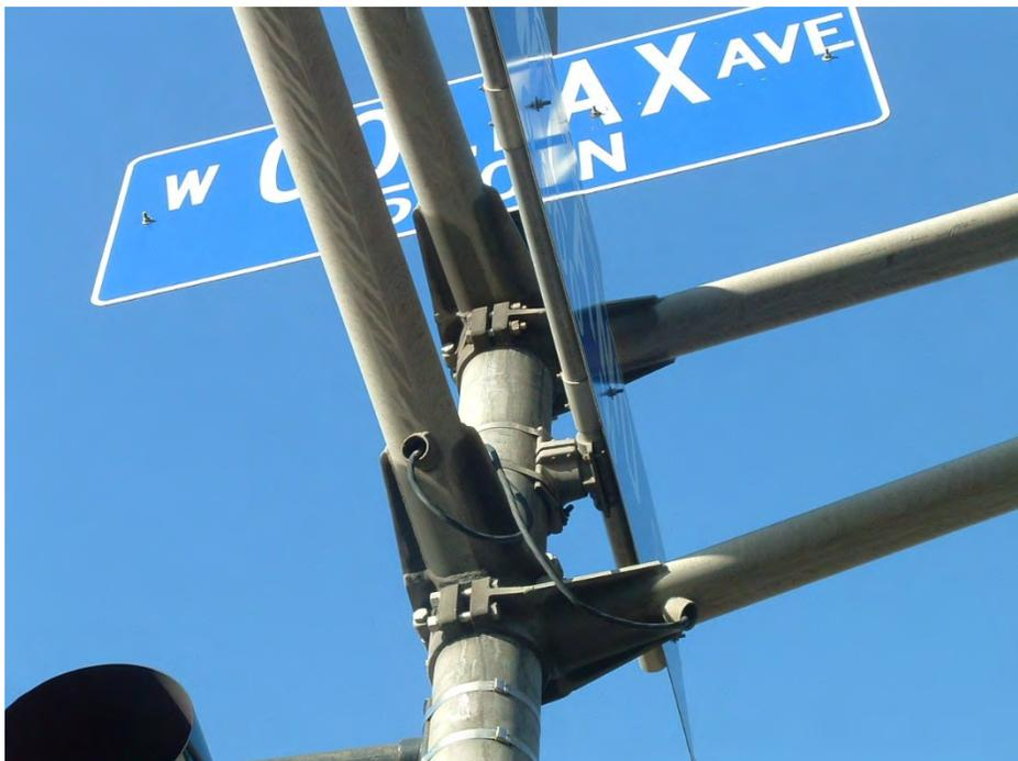
**Type 109:** Quad arm, clamped connection
