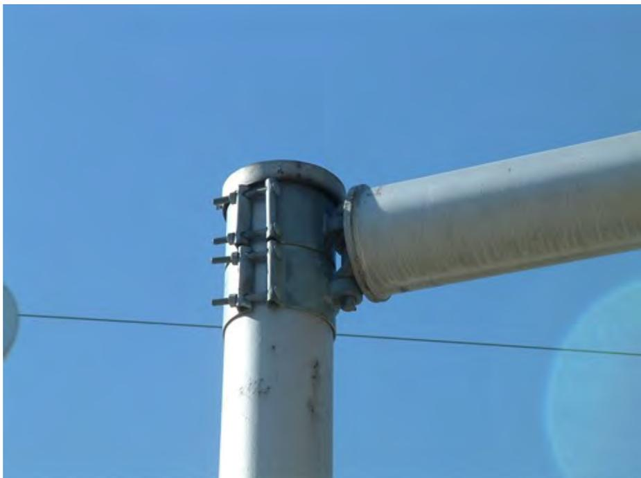
**Type 028:** Single arm, double collar connection, or double U-bolt connection
