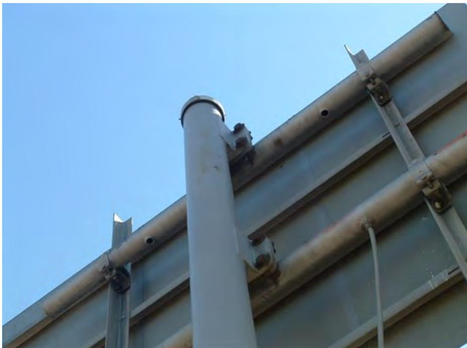
**Type 049:** Double arm, horizontal bolted connection to simplex plate on front of pole
