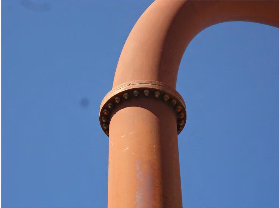
**Type 039:** Monotube, vertical bolted connection, no stiffeners
