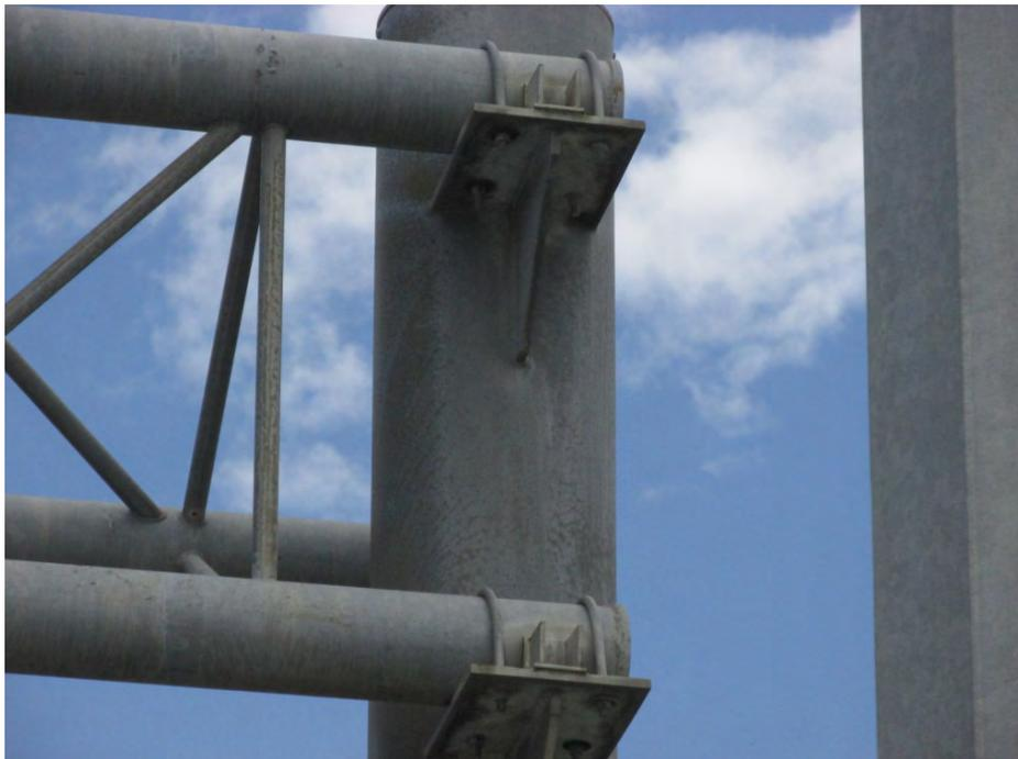
**Type 011:** Three arm truss, U-bolt fitted connection on bearing plates
