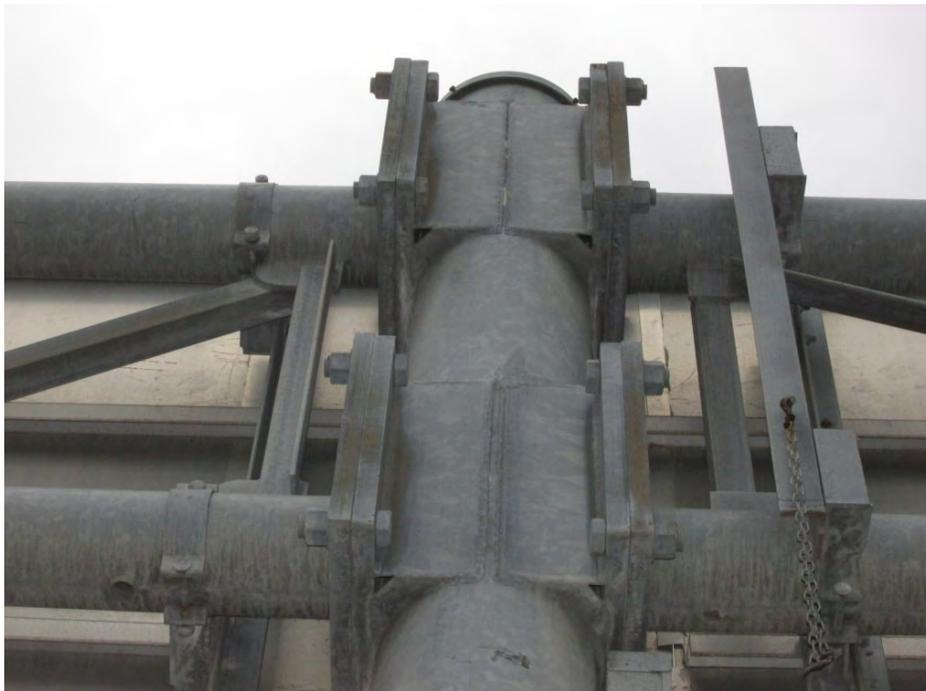
**Type 036:** Single face sign, double arm, double horizontal bolted connection to simplex plate
