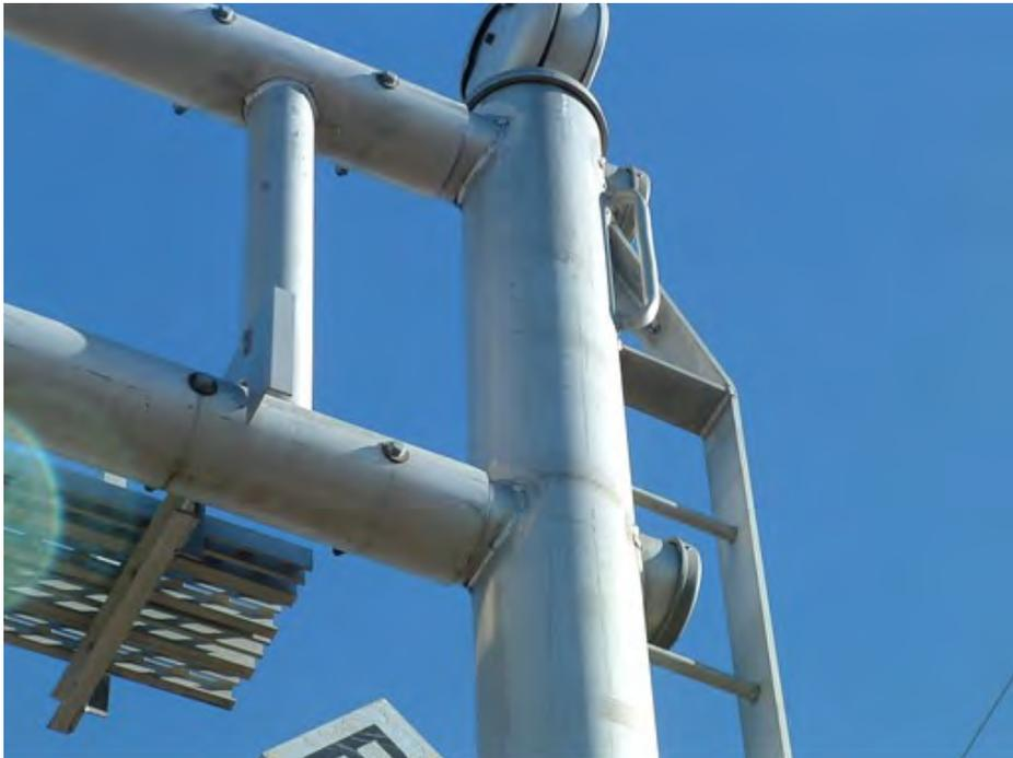
**Type 058:** Double arm, pipe fitted through vertical, welded
