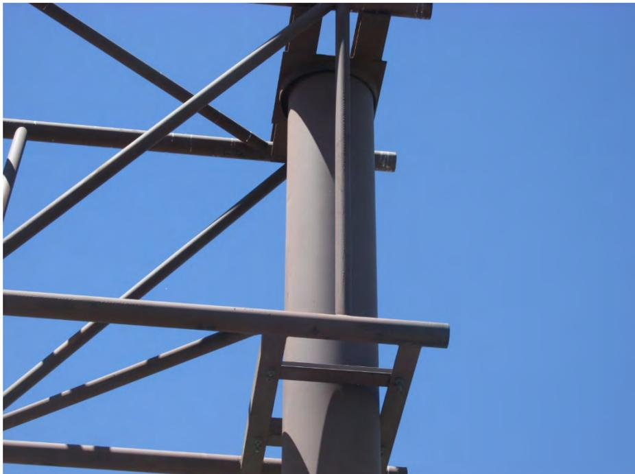
**Type 016:** Double arm (pipe) truss, cap connection
