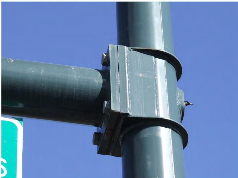
**Type 111:** Single arm, 4 bolt connection to simplex plate with welded bracket stiffener
