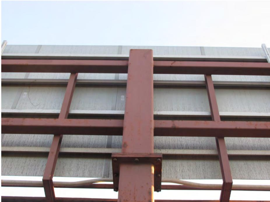
**Type 005:** Double arm, square column, vertical bolted connection
