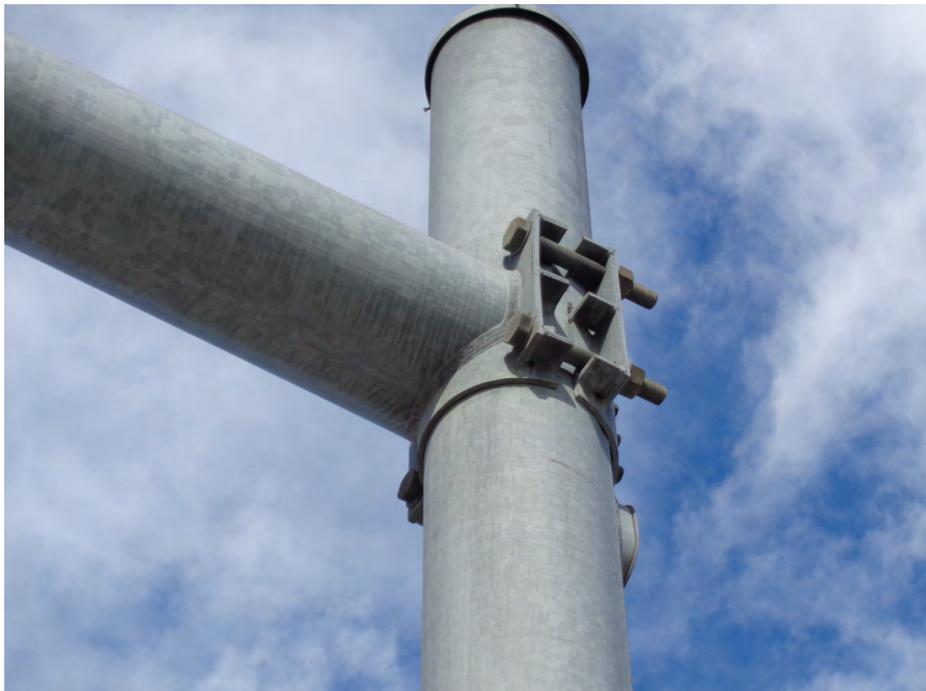
**Type 105:** Single arm, welded-clamped connection
