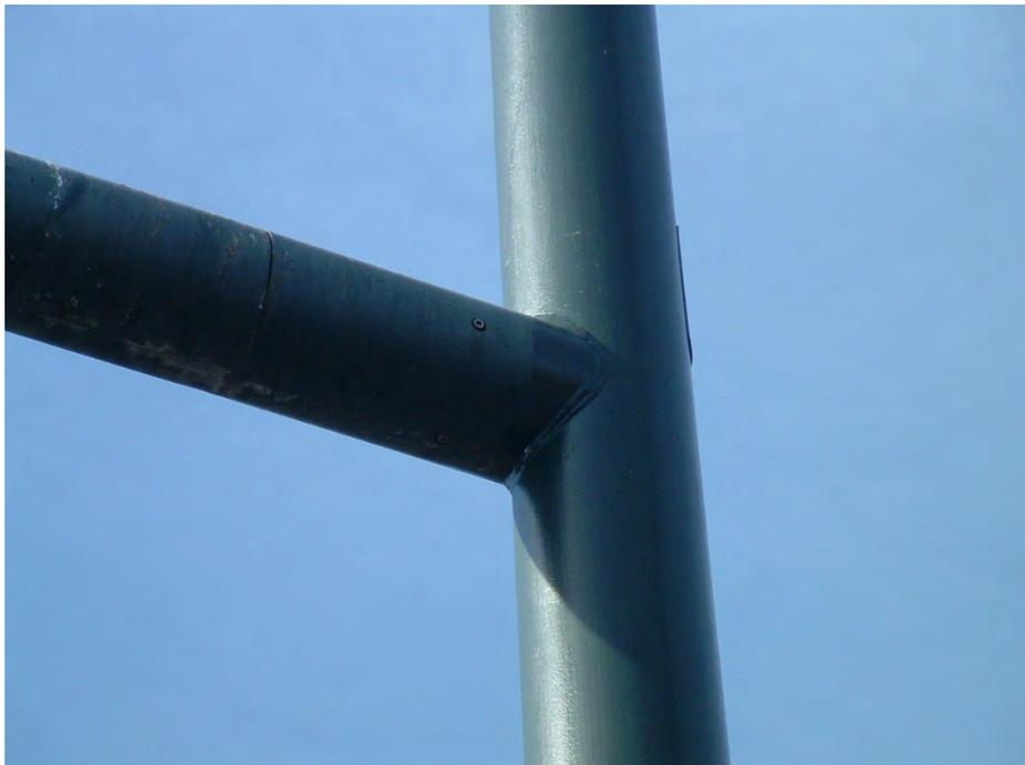
**Type 113:** Single arm, circular welded connection
