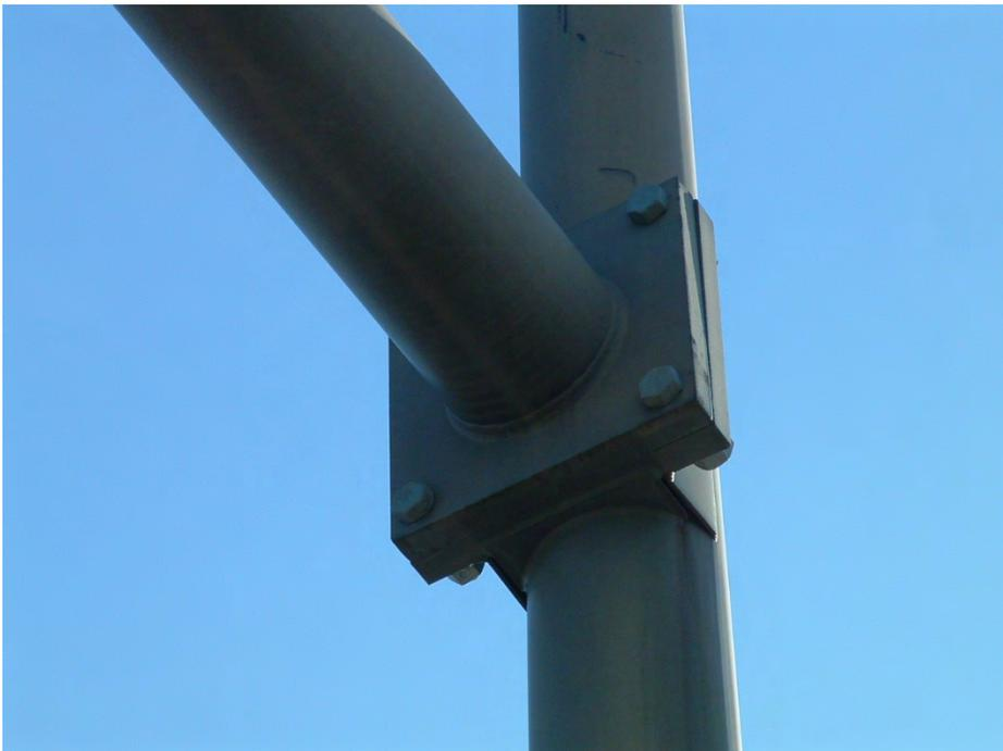
**Type 107:** Single arm, 4 bolt connection to wide simplex plate
