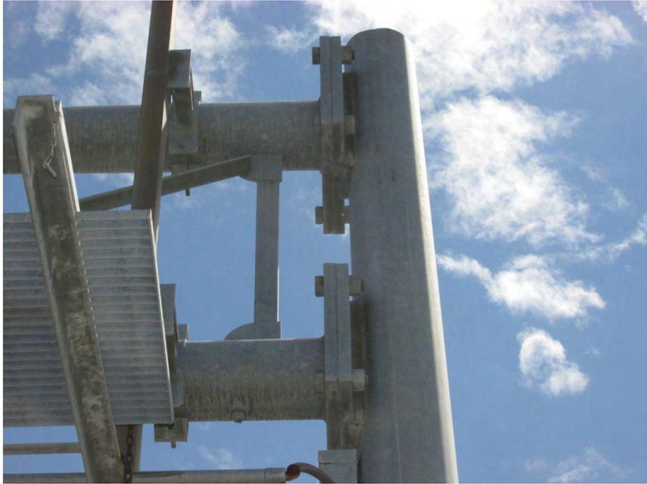
**Type 045:** Double arm, horizontal bolted connection to plate
