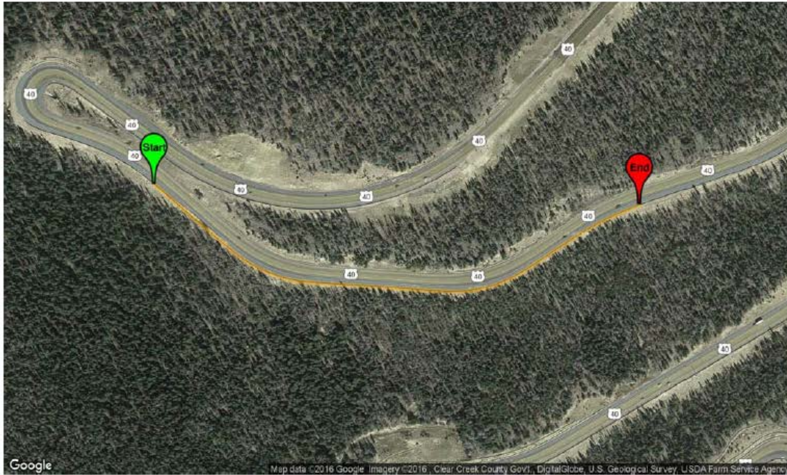
Overview of Wall R040A244649RRA on CDOT Route 040A
