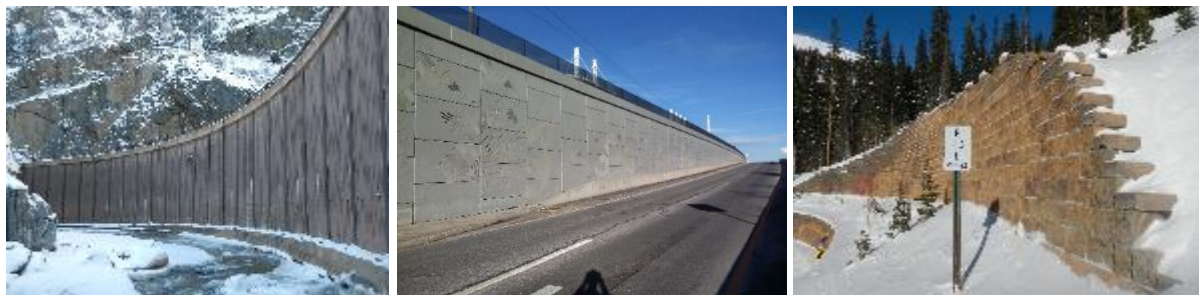
Common Examples of Retaining Walls Found in Colorado
