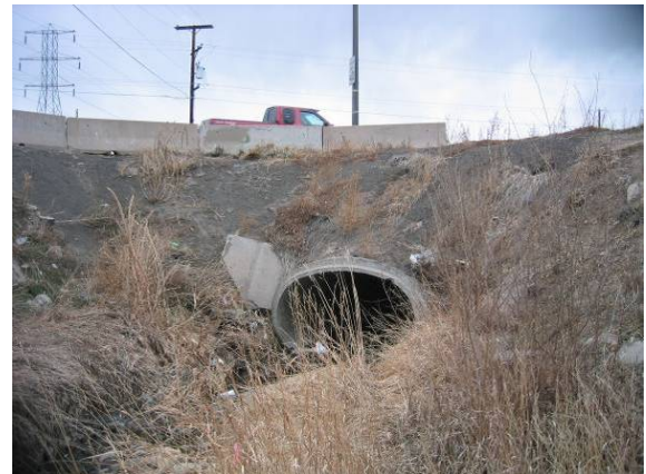
52 EXHIBIT 5-4: DRY GULCH CULVERT
