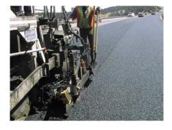
placement of asphalt rubber. To ensure the highest quality, the placement temperatures must be 65 degrees and rising. This makes night paving in Colorado virtually impossible. Since traffic congestion requires most construction in Colorado, especially in urban areas such as Denver and Colorado Springs, to be conducted at night, there is a very small window of opportunity to pave.
