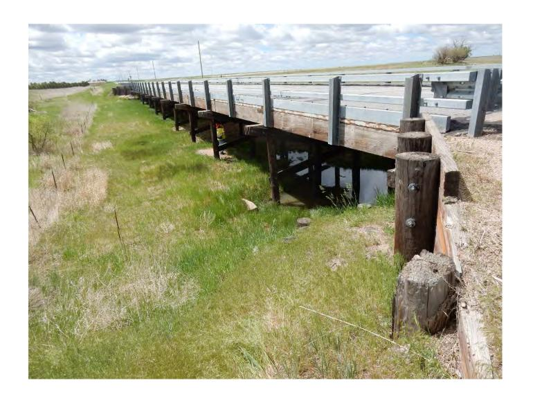
Sandy Creek Bridge, Phillips County, State Highway 59, Treated Timber Stringer with metal plank deck
