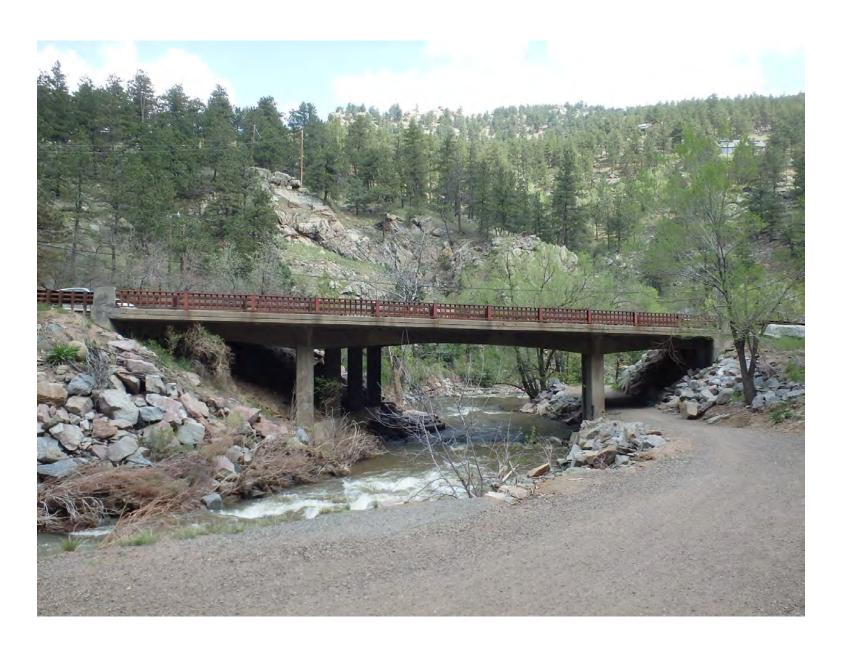
Boulder Creek Bridge, Boulder County, State Highway 119, Concrete Slab and Girder Continuous
