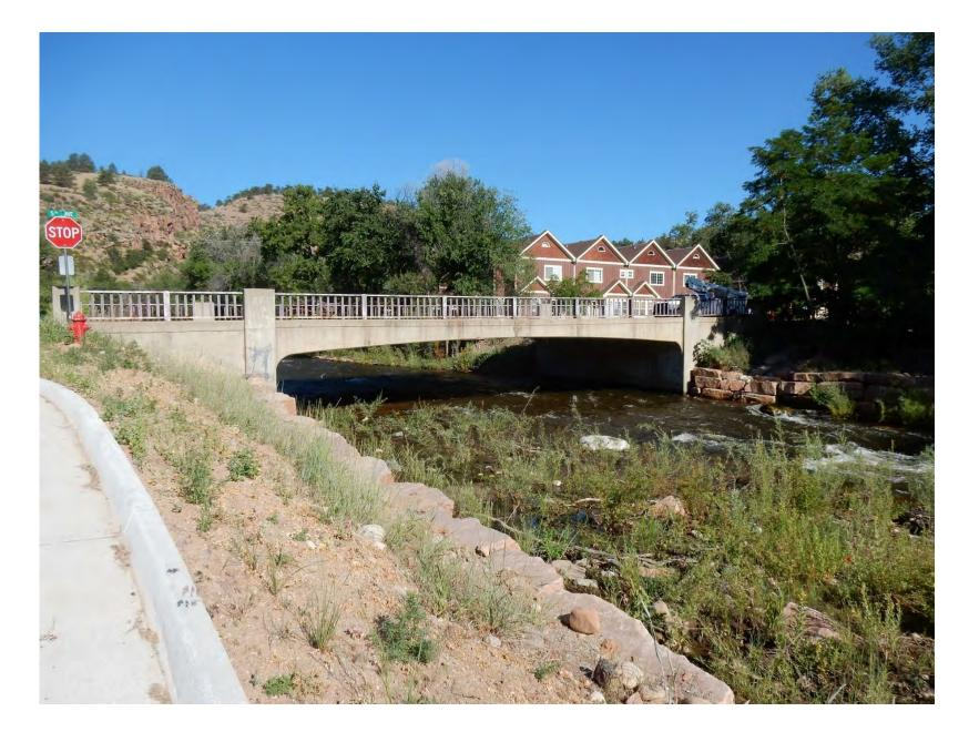
North St Vrain Creek Bridge, Boulder County, State HIghway 7, Concrete Rigid Frame
