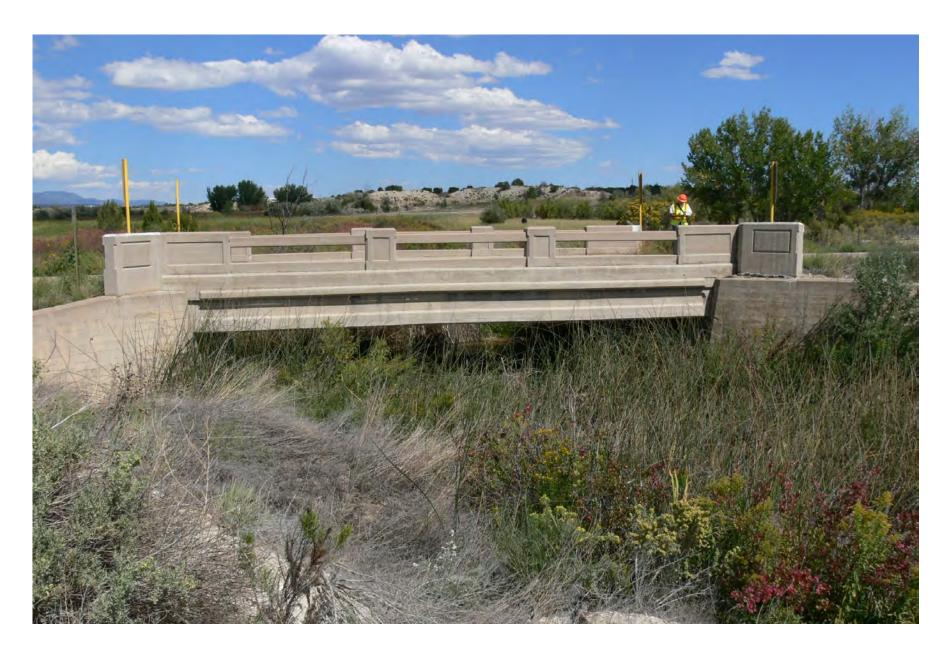
No Name, Fremont County, State Highway 120, Concrete slab and girder
