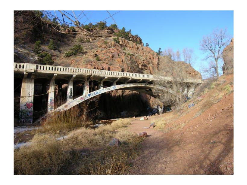
Fountain Creek Bridge, El Paso County, US Highway 24, Concrete Two Rib Open Spandrel Arch
