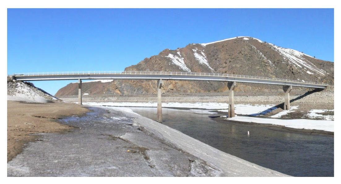
Blue Mesa Reservoir Bridge, Gunnison County, State Highway 149, Welded Girder Continuous and Composite
