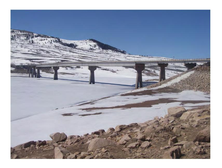
Blue Mesa Reservoir Bridge, Gunnison County, US Highway 50, Welded Girder Continuous and Composite
