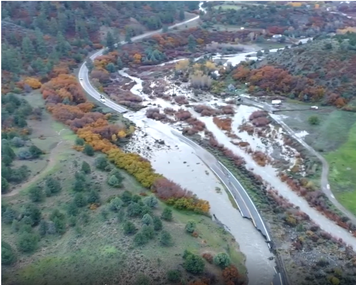
Highway destroyed by flood on CO 151 at MP 27
