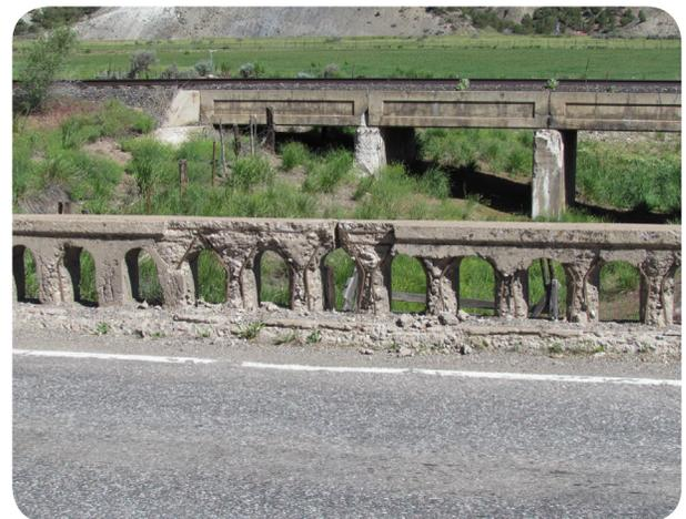
Image 5. Deterioration of the Deck on US 6 over Castle Creek in Eagle County (F-09-K)
