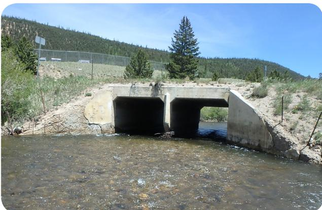
Image 1. Deterioration of West Wing Walls on SH 9 over Platte Gulch in Park County (G-12-C)
