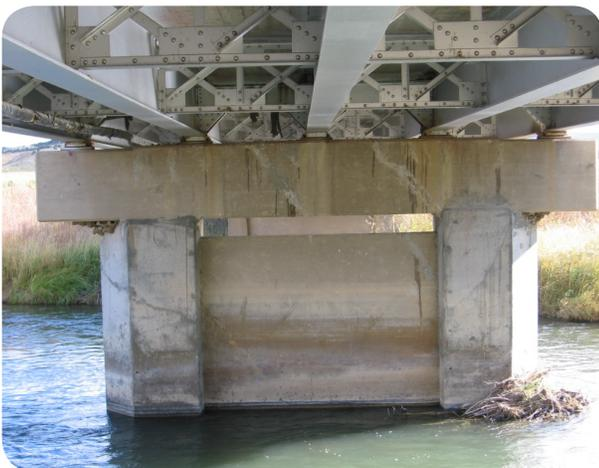
Image 4. Deterioration of the Substructure on SH 64 over White River in Rio Blanco county (D-03-A)
