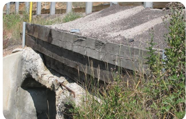
Image 2. Deterioration of Concrete on US 24 over Draw in Teller County (I-15-AO)
