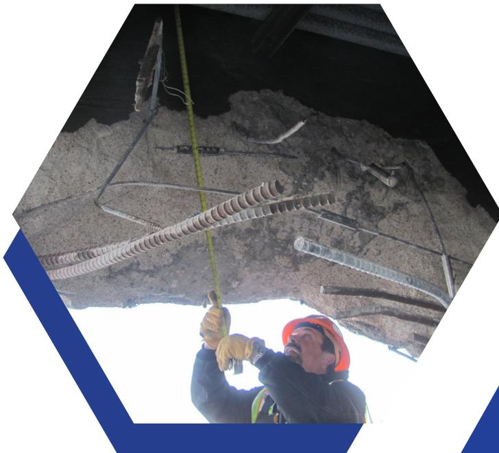
Image 10. Impact Damage from Truck Strike Speer Blvd over I-25 in Denver (E-16-EW)
