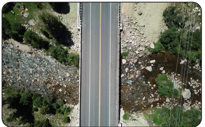
Image 4. Completed Structure US 34 over N Fork Colorado River in Grand County Aerial View (D-13-A)
