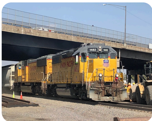
Image 12. Train Switch onto the New UPRR over I-70 bridge
