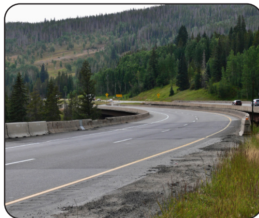
Image 17. I-70 over Polk Creek in Eagle County (F-12-AS)
