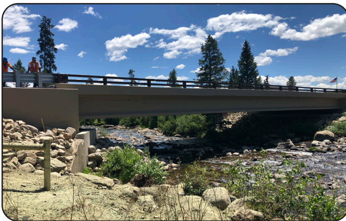
Image 3. Completed Structure US 34 over N Fork Colorado River in Grand County (D-13-A)
