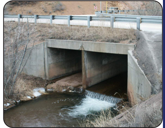
Image 13. US 24 Service Rd over Fountain Creek in El Paso County (I-17-X)
