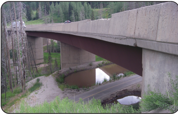
Image 1. I-70 over Polk Creek in Eagle County (F-12-AS)
