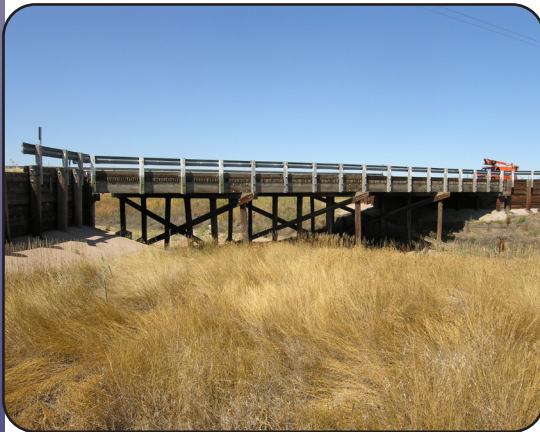
Image 14. SH 61 over Surveyor Creek in Washington County (D-25-E)
