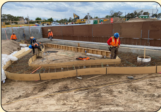
Image 14. Wall footing for the Swansea Park Playground
