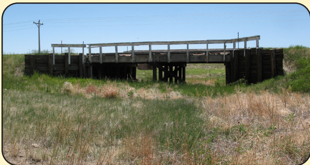
Image 17. I-70 Service RD over Draw in Arapahoe County (F-20-L)
