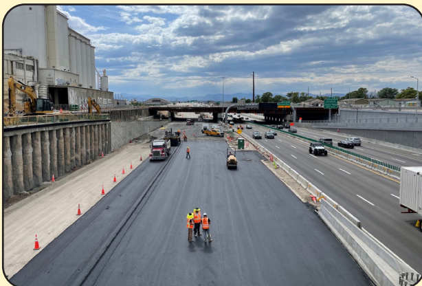
Image 15. EB I-70 Lowered Section Paving
