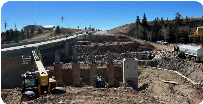
Image 22. Recently Installed Caissons for the Future Bridge
