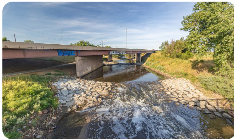
Image 17 & 18. Constructed Drop Structures to Mitigate Scour on I-76 over Clear Creek (E-16-LT/LU)
