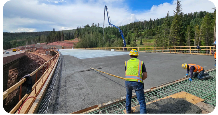
Image 8. New Bridge Deck of the future I-70 WB over Polk Creek
