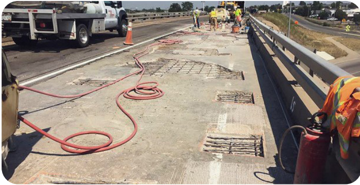
Image 21. Emergency Repairs on I-270
