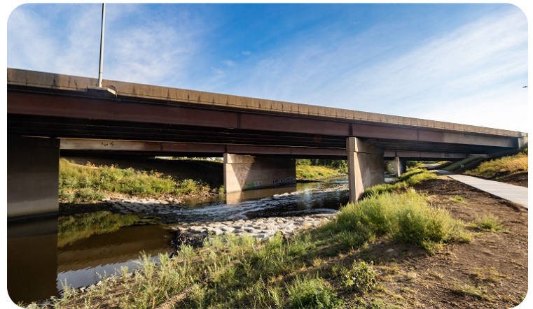
Image 17 & 18. Constructed Drop Structures to Mitigate Scour on I-76 over Clear Creek (E-16-LT/LU)
